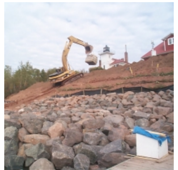
Shoreline Stabilization work in 2002
