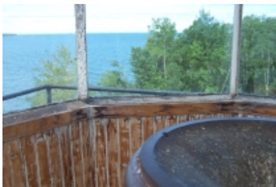
Restoring the tower, repainting interior and exterior walls, and repairing a cracked foundation are just a few of the tasks included in this rehabilitation of the Raspberry Lighthouse.
