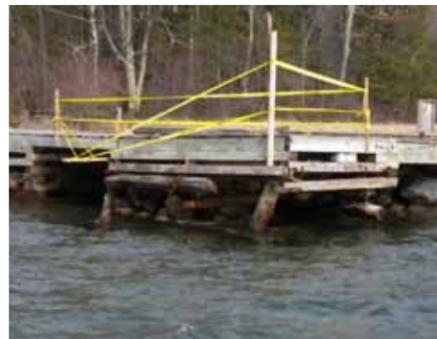
Ice damage to the dock at Otter Island has forced sections of the dock to be closed pending repairs.
