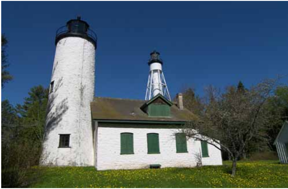
Work at the Michigan Island Light Station will include four buildings and clearing four acres at the site to restore the cultural landscape.
