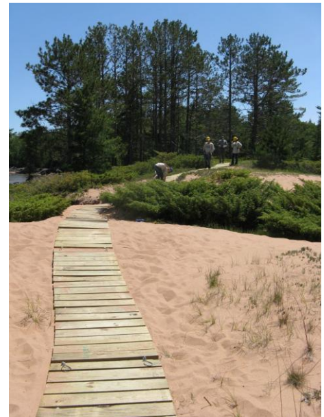
New floating boardwalk at Stockton Julian Bay
