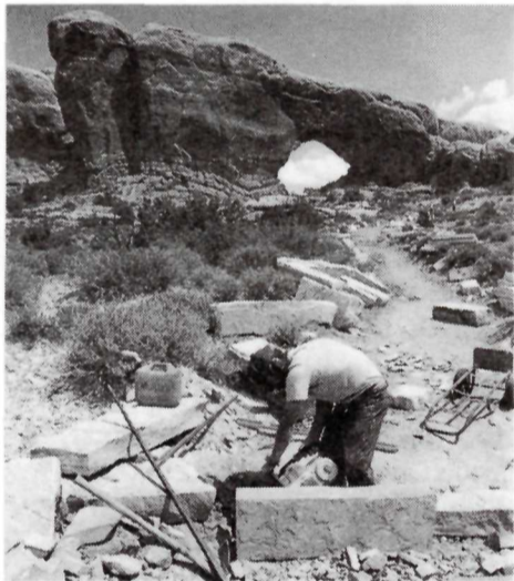
Trail work at North Window.
