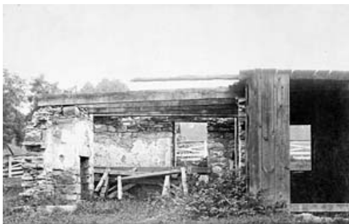
The stone building in ruins. The western wall of the north room is collapsed, revealing the warming fireplace. The south room has a rough wooden roof and western wall.
