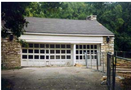
The stone building rebuilt as a garage.
