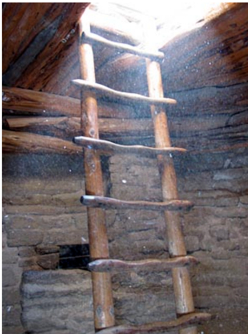
Ladder and beams in a kiva at Spruce Tree House, Mesa Verde. Photo by Ranger Kathryn
