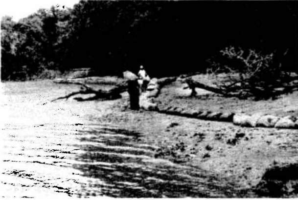
Shoreline stabilization test area, Cumberland Island National Seashore—placing shell rake, Cumberland Island, GA. (Photos courtesy Robert M. Thorne.)
