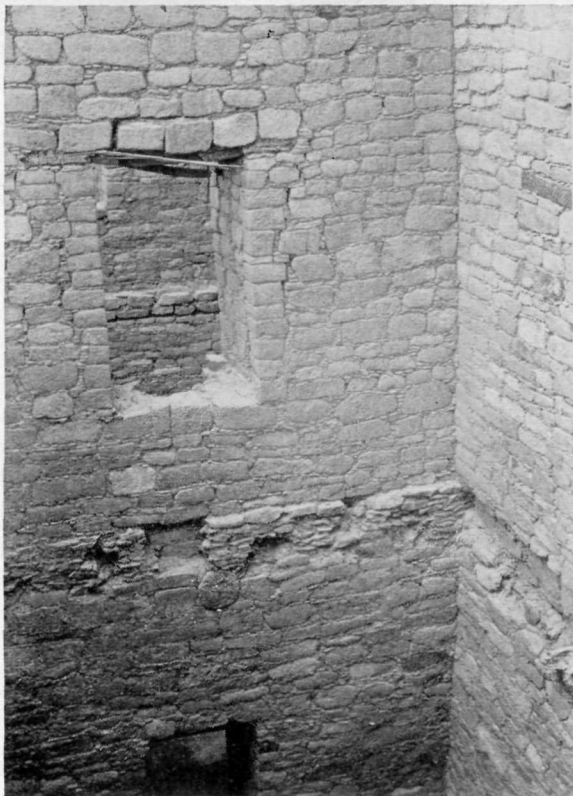
A section of two-story wall showing the doors with wooden lintels in place. The irregular line between the doors was where the floor of the second story began.
