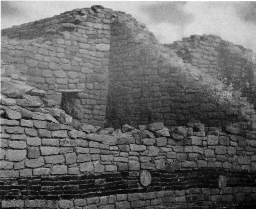
Masonry of the main ruin, showing decorative inlay band of dark stones.
