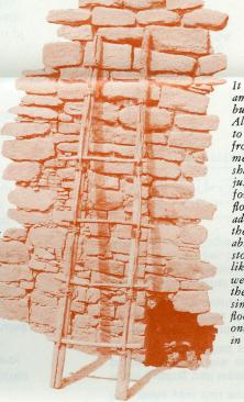
It took a tremendous amount of labor to build these walls. All of the stones had to be carried here from several kilometers away, then shaped by hand with just another stone for a tool. As the floors and walls were added above ground. the builders probably hauled the stones up on ladders like this one. Ladders were also used by the Pueblo Indians simply to get from floor to floor. This is one of six found in the ruins.
