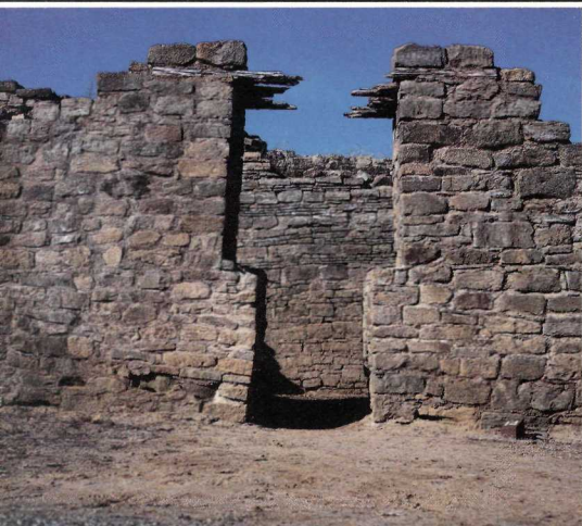
This T-shaped doorway in the West Ruin is Mesa Verdean in origin; the far wall is Chacoan in construction.
