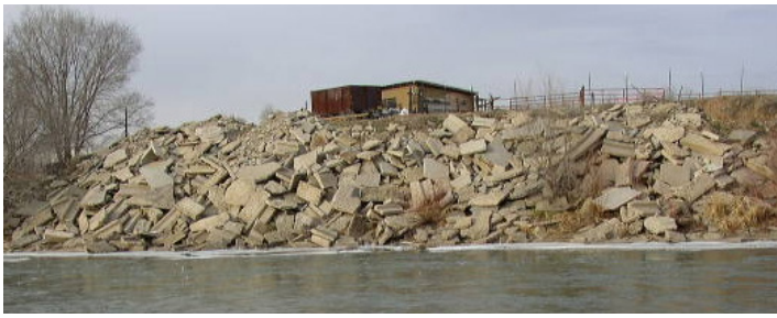
Figure 16. Photograph of rip-rap along the Animas River. The steepest section of bank along the Animas River at Aztec Ruins National Monument is located along this property, which the National Park Service acquired in 2009. This photograph was taken in 2004. Since then, the National Park Service has removed the shed and fencing, but the rip-rap remains. National Park Service photograph by Kim Johnson.
