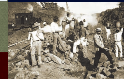
Workers pause during construction of a "cut" through terrain for the Panama Canal, 1913.
