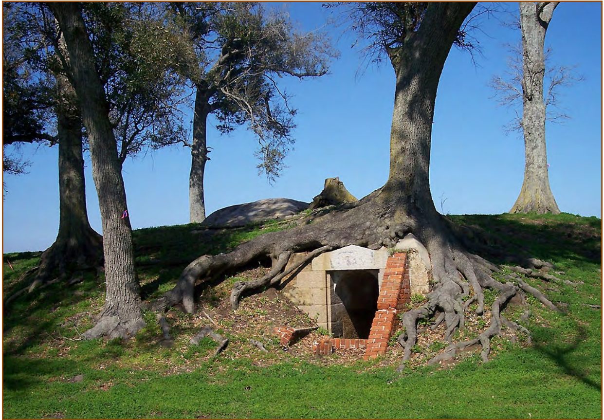
Figure 4. Natural threats endanger many battlefield features in Louisiana. Here, the parapet and bombproof at Fort Jackson are overgrown with mature trees. Root systems will slowly break apart the masonry and, if the trees blow over in a storm, dislodge chunks of parapet. Photograph by Joseph E. Brent, 2008.
