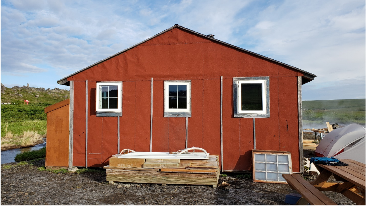
Photo 3: Serpentine Hot Springs Bunkhouse, Gable End, Toward Northwest, BELA Files, 2018
