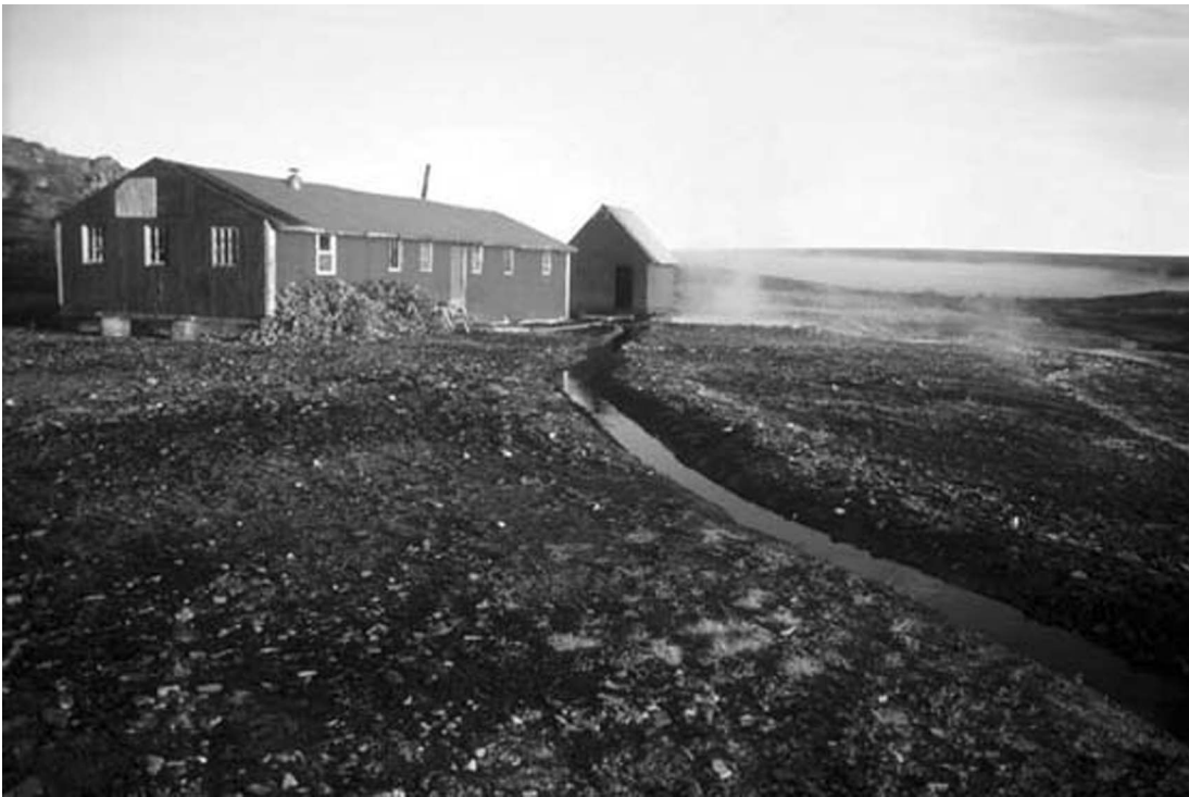
Figure 4: Cold water diversion ditch and bermed pool (no longer extant), pre-1996, with Bunkhouse and Bathhouse in background, CLI Program Files
