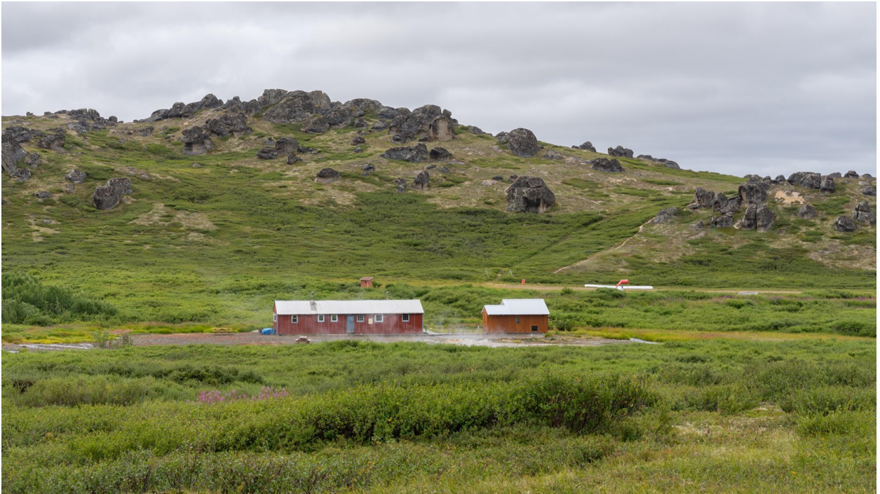
Photo 1: Overview of facilities at Serpentine Hot Springs, Bunkhouse, Bathhouse, Privy, Airstrip, Toward Southeast, BELA Files, 2017
