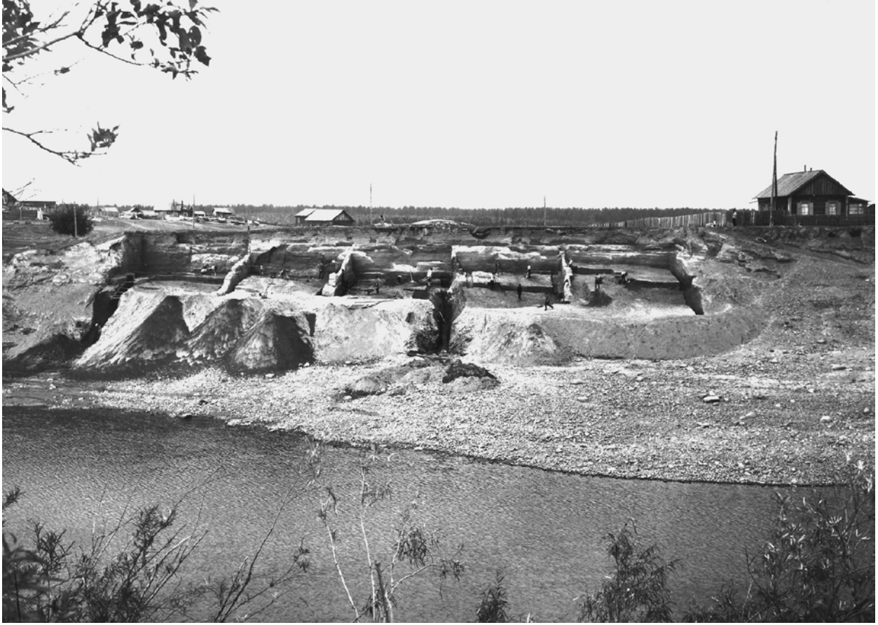
Figure 19. View to the excavation of the Bel'kachi I site.
