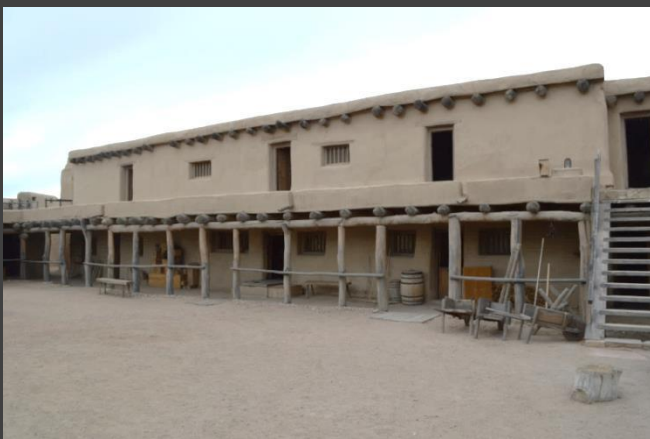
Tom Long, West Side of Fort, Taken 02/29/2016
