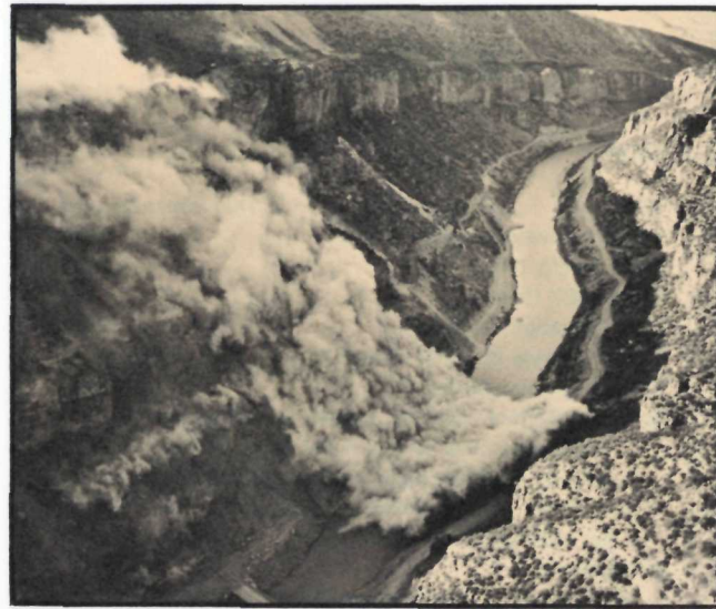
Blasting loose rock from canyon walls prior to start of construction
