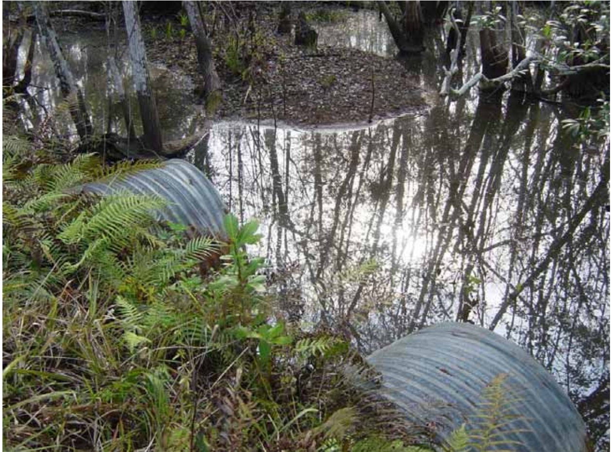
Figure 7. Intact culverts along an access road within Big Cypress National Preserve. Photo is taken from the road. Note the height of the road above the water level and the degree of ponding behind the roadway. Photograph by Trista L. Thornberry-Ehrlich (Colorado State University).
