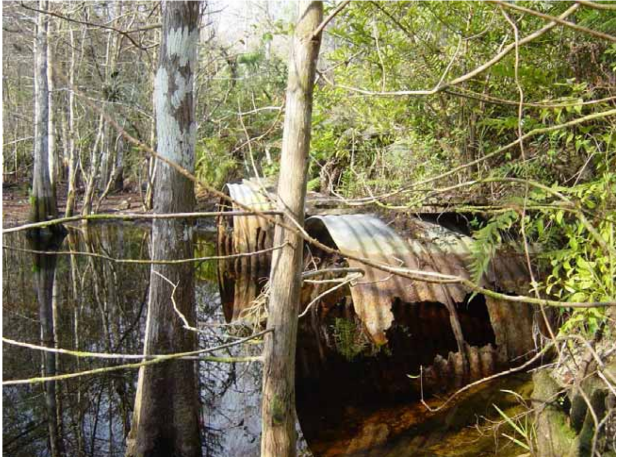
Figure 6. Rusting culvert along an access road to an oil pad at Big Cypress National Preserve. Photograph by Trista L. Thornberry-Ehrlich (Colorado State University).
