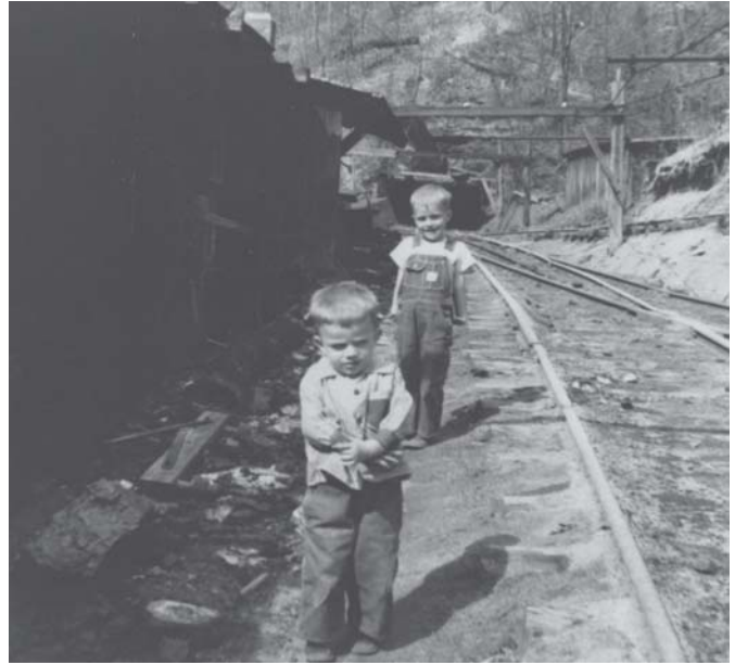
Rail tracks leading into Mine 18
