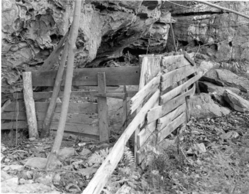
Figure 1 Hog pen built into cliffside west of barn
