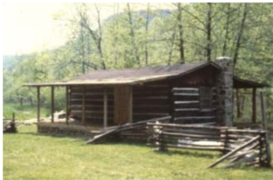
One of the guest cabins at Charit Creek Lodge.
