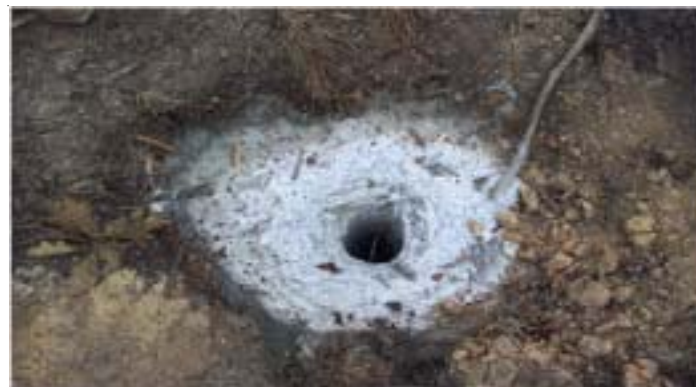
Well casing hole plugged with concrete. NPS Photo.
