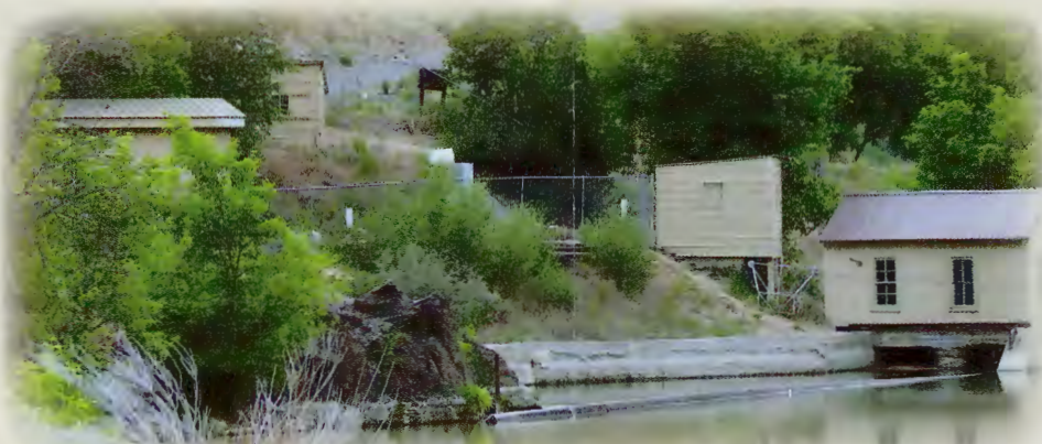
Gate and equipment houses provide for the workings of the tunnel at East Portal.
