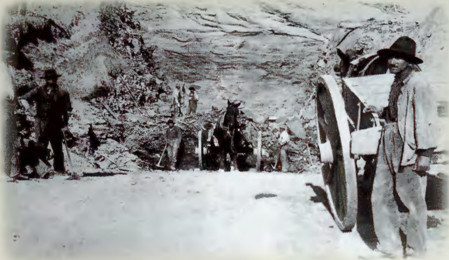
While digging continued on the tunnel, a massive effort was made to extend a system of ditches to carry the water to individual farm fields. The largest of these, the South Canal, would carry water from the tunnel to the Uncompahgre River.
