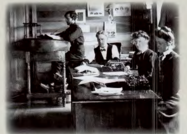
While work progressed around the clock in the tunnel, office help continued to keep the laborers supplied. Payroll, purchasing and repairs on equipment were all part of the effort.
