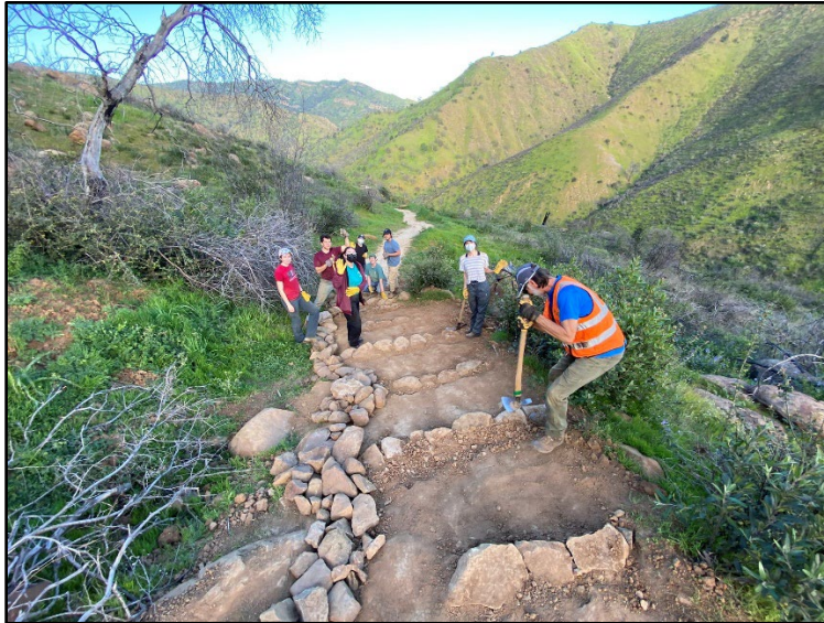
Credit: UC Davis Reserves. Youth volunteers working on trail construction.
