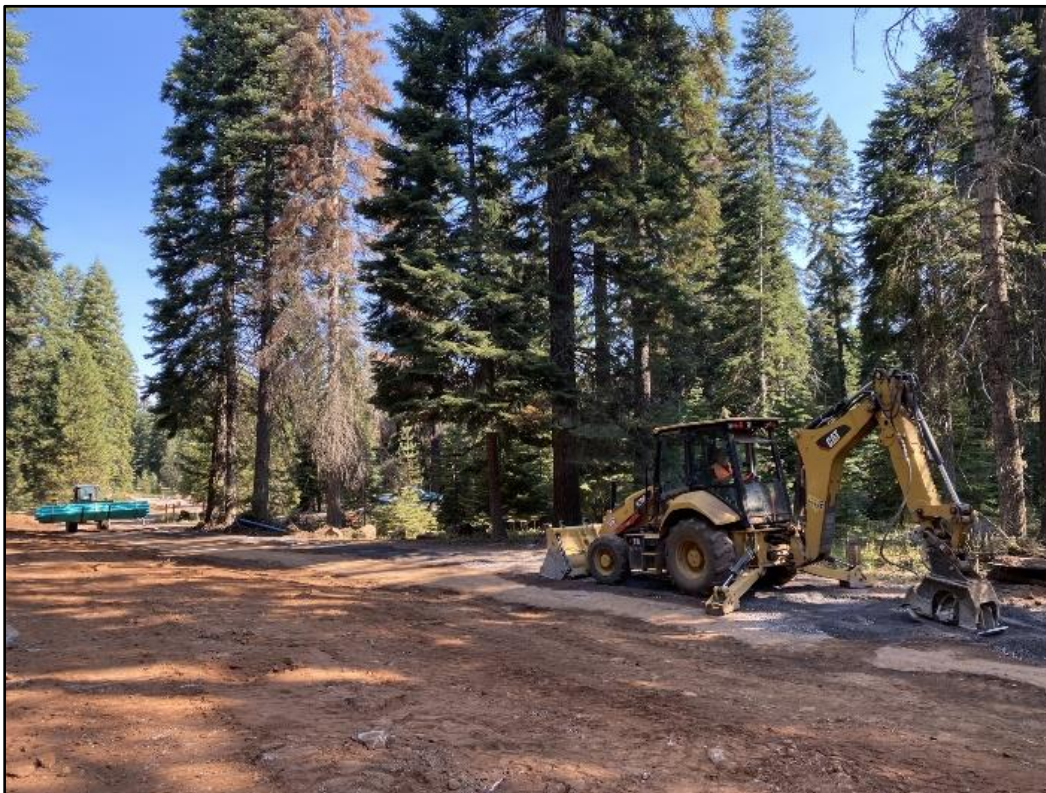
FY 2023 infrastructure repair work in Hyatt Lake Campground
