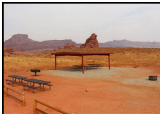
Figure 9. Group campground facilities with wooden post fencing barrier; the Ledge, Utah.
