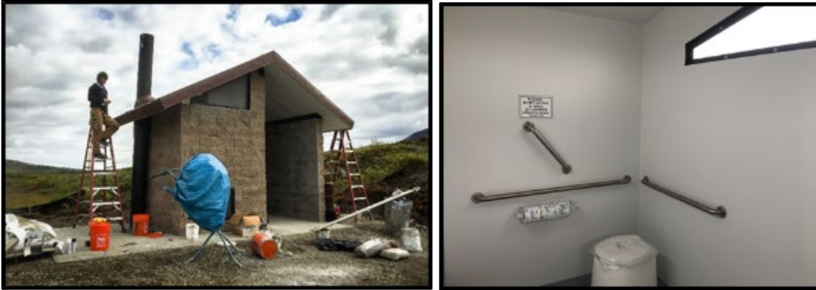
Figure 4. Single “unisex” vault toilet.
