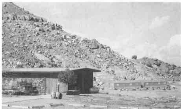
Figure 44. Buildings erected by the Bureau of Land Management. The Visitors Center, with exhibits, is in the foreground. Two metal buildings, erected over the bone bed are on the right. These are intended to protect the deposit and to allow visitors to view excavations in progress.
