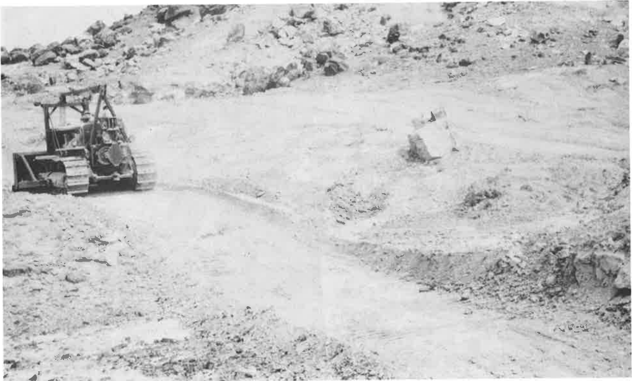
Figure 30. Bulldozer covering the quarry site. This operation was carried out yearly to lessen the possibility of vandalism. There were no known damages by souvenir hunters during the entire period of operations.
