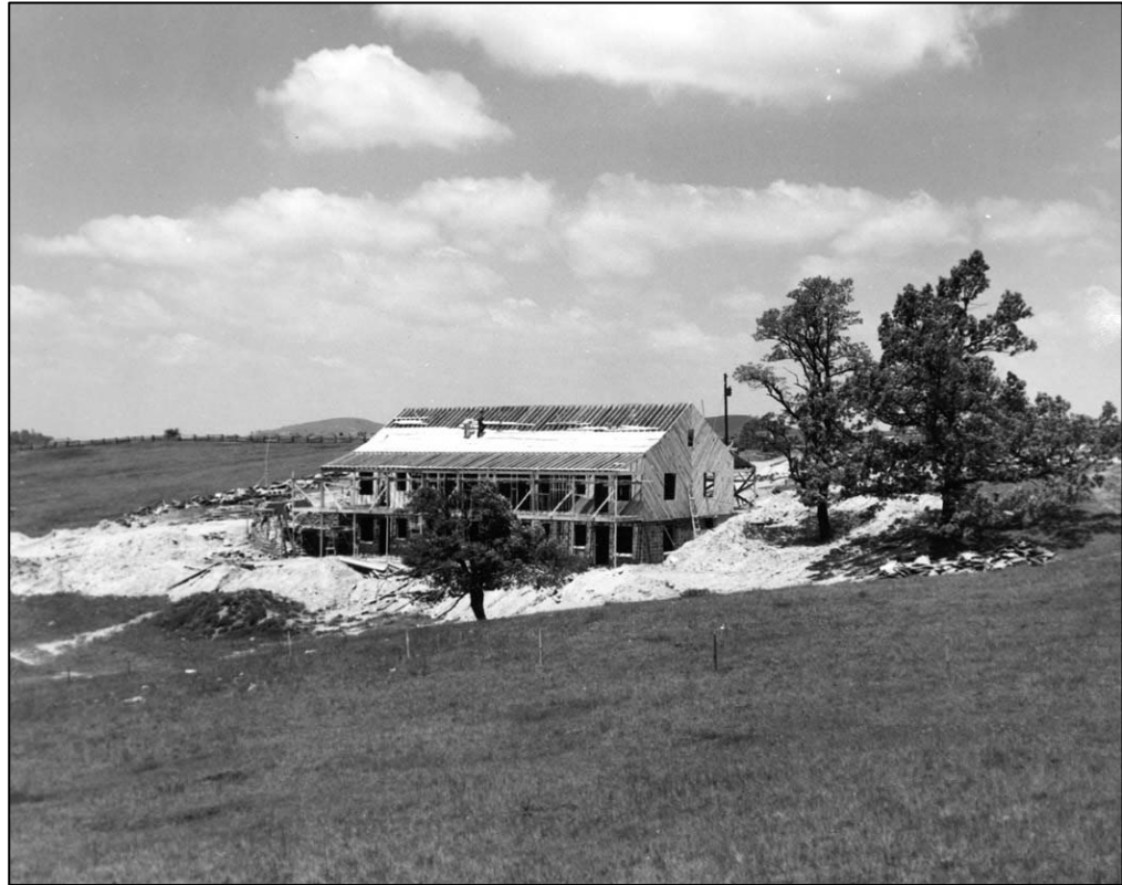
Fig 8-15. Bluffs Lodge during construction circa 1949
