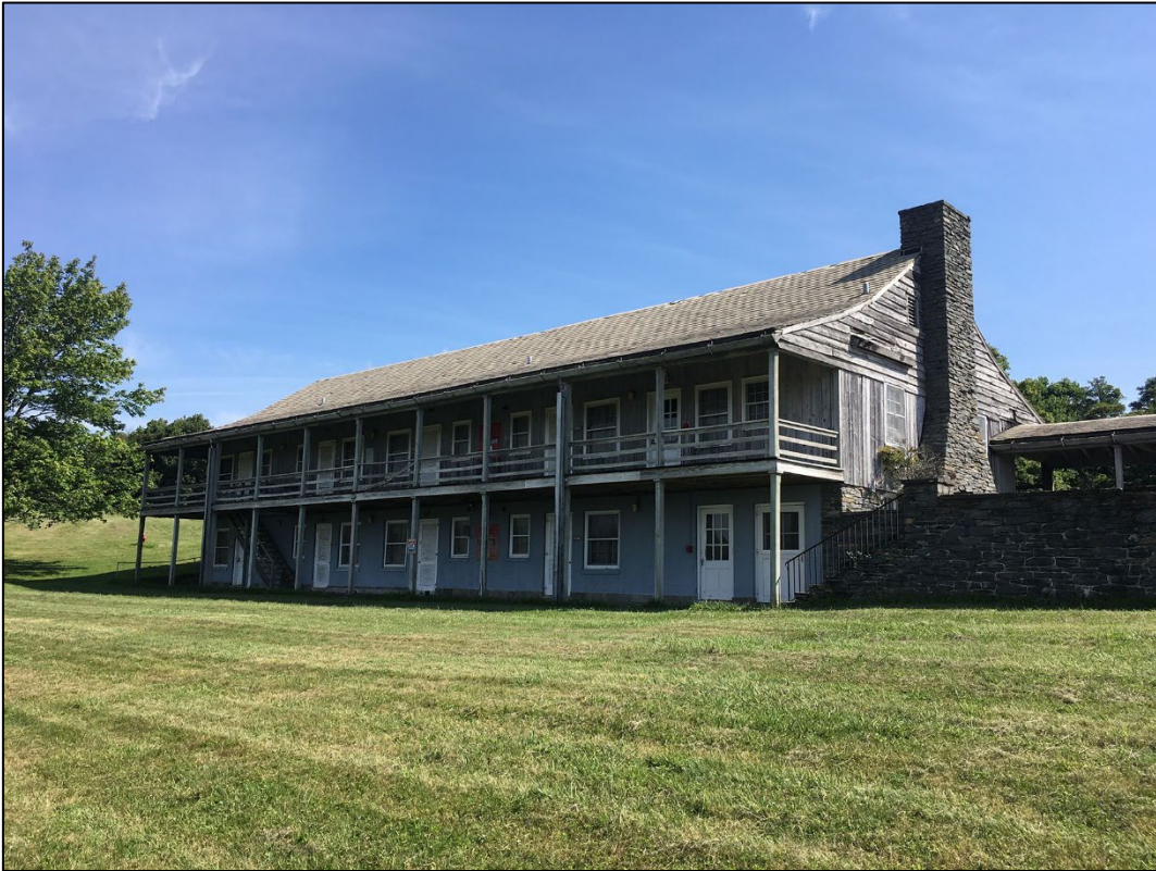
Fig 8-1. View of Bluffs Lodge, south façade, illustrating interplay with surrounding topography, facing north (2021)
