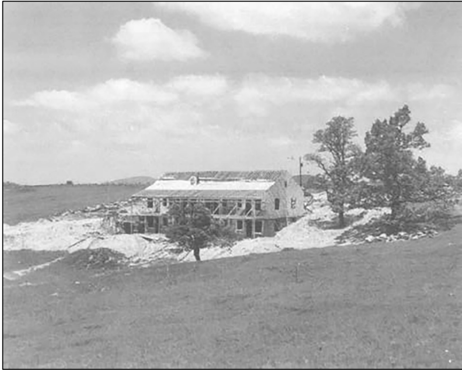
Fig 6-8. Construction of Bluffs Lodge, c. 1949, (Orig. Photo not located, provided by SERO from Bluffs Lodge CLI files).
