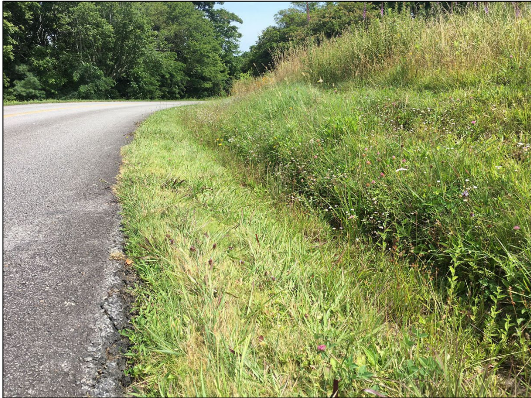
Fig 8-25. Close-up of stone gutter along Bluffs Lodge entrance road. Heavily obscured by overgrown vegetation and accumulated debris. Facing northwest (2021)
