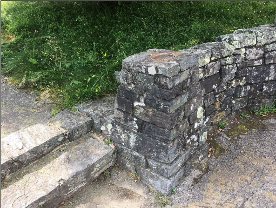
Fig 8-30. Rustic-style stone drinking fountain incorporated into Robert L. Doughton Memorial wall (2021)
