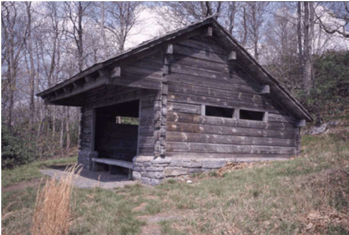
Trail Shelter, Building # 103 (2002).
