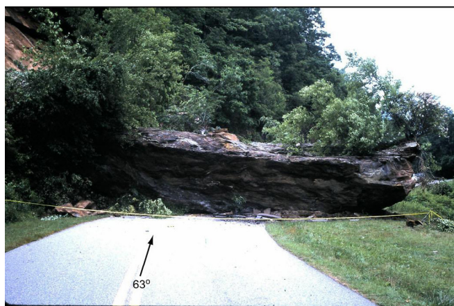
Figure 27. Photograph of huge rockfall blocking the Blue Ridge Parkway. On 15 June 1999, a rockslide covered the parkway, causing its closure for several days. The rock is metagraywacke from the Alligator Back Formation (Zabg) near Crabtree Meadows. Arrow and azimuth, which are part of original graphic, indicate direction N63°E. Graphic is part of photomosaic CER-001 from Mersch et al. (2008a).
