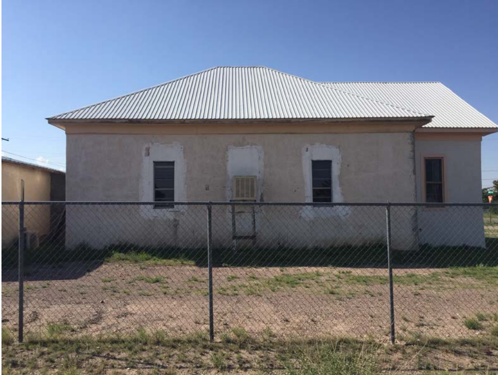
Photo 5: South elevation showing 1909 schoolhouse, looking north. (June 14, 2019)
