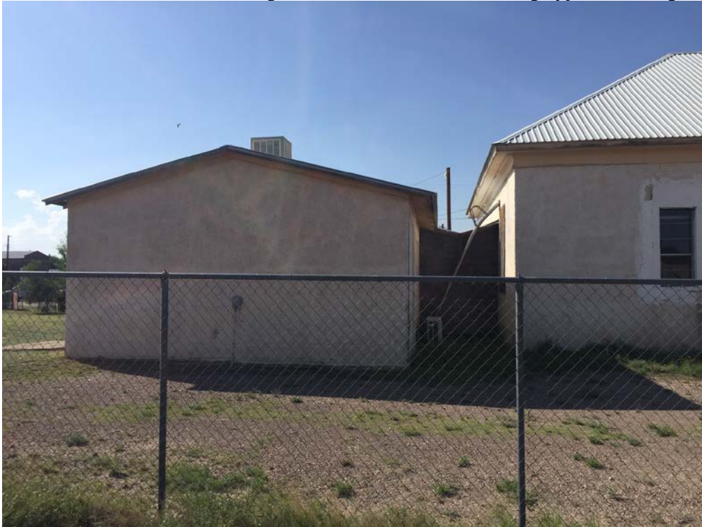
Photo 6: South elevation showing 1927 Band Hall and connecting hyphen, looking north. (June 14, 2019)
