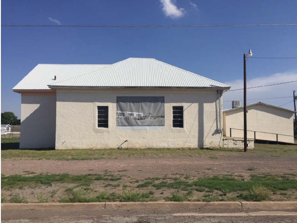
Photo 3: North elevation of 1909 schoolhouse, looking south. (June 14, 2019)
