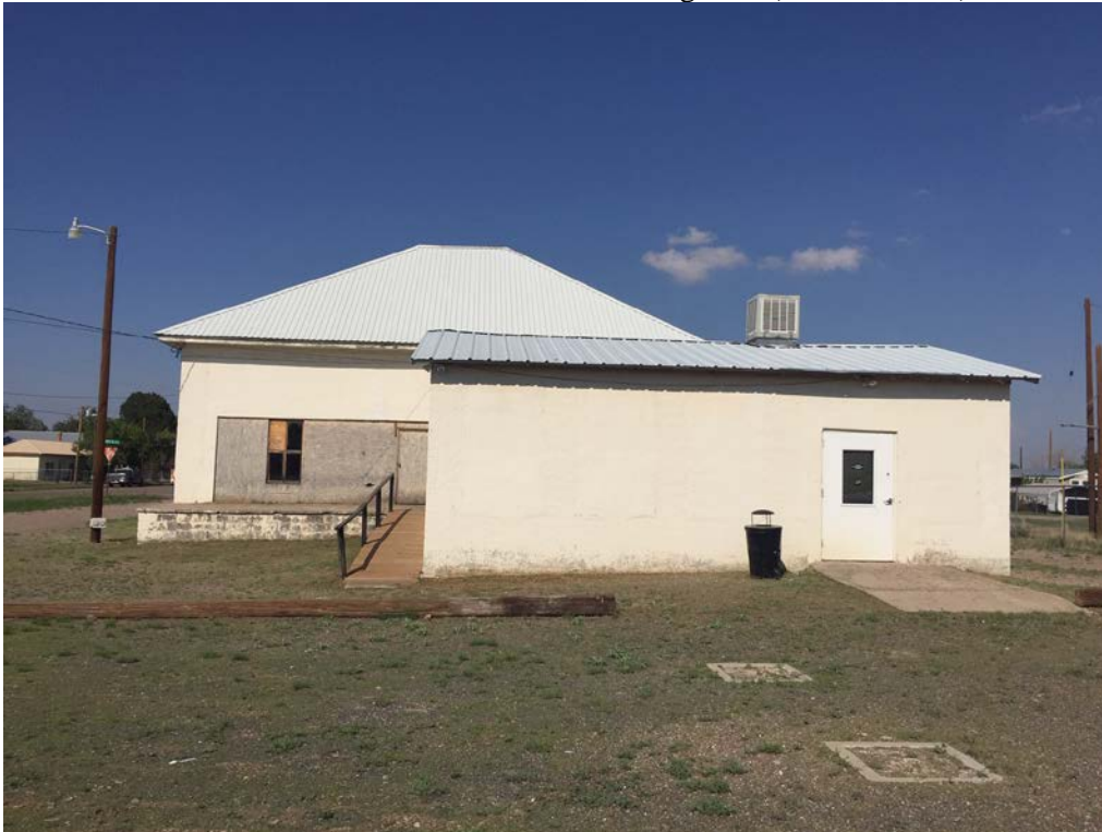
Photo 4: West elevation of 1909 schoolhouse, looking east. (June 14, 2019)
