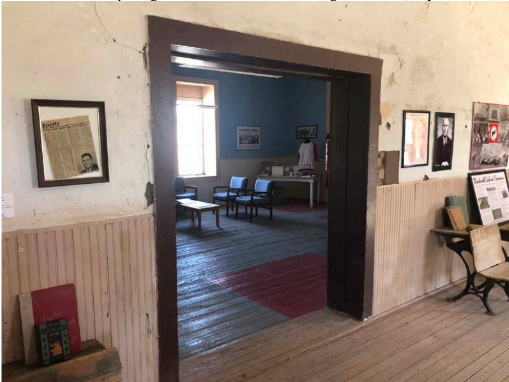
Photo 10: Interior opening between classrooms. Looking northeast. (May 18, 2019)
