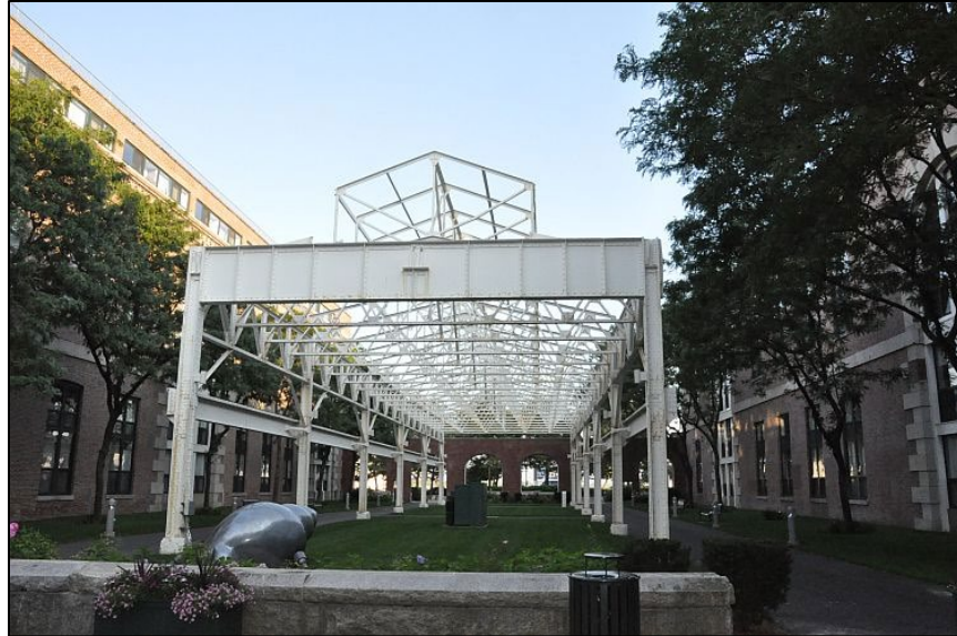
Figure 2-4. Example Open Frame Structure (Parris Landing, Building 42 at the Charlestown Navy Yard)
