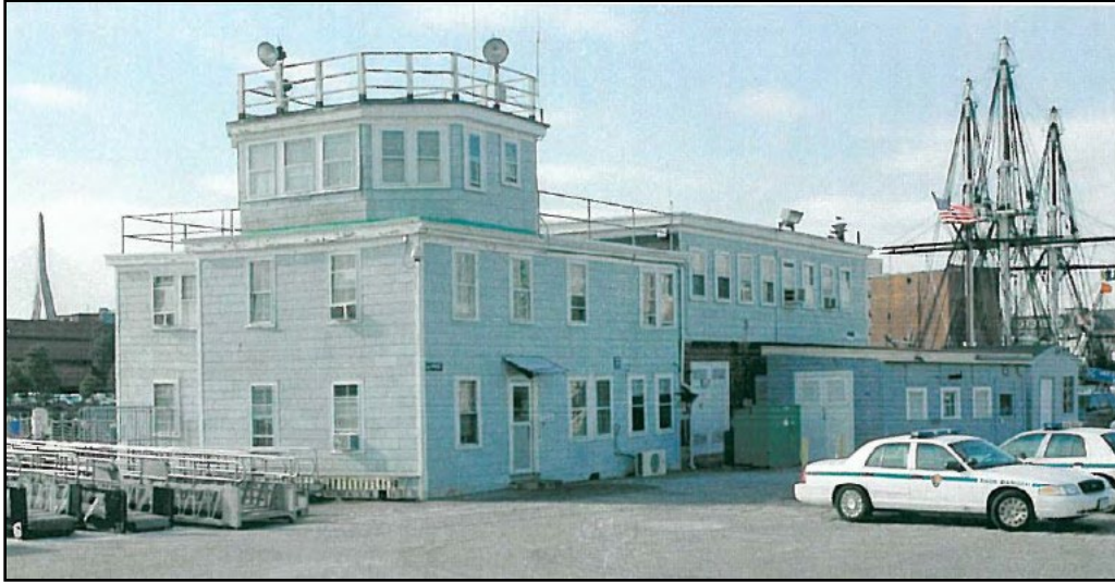
Figure 3-5. Building 109 Looking Northwest from Pier 1
