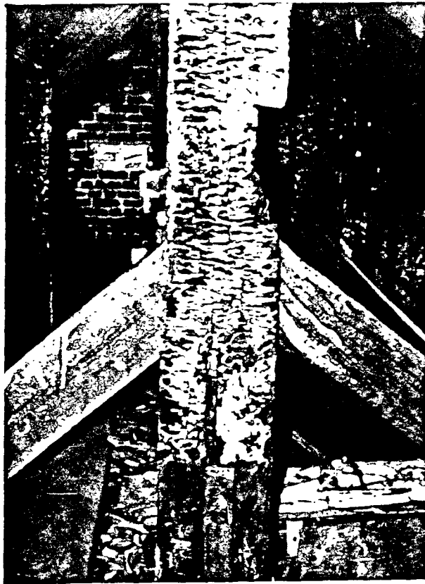
ILLUSTRATION 46. OLD STATE HOUSE: NOTCH IN TRUSS KING POST, 1987.
