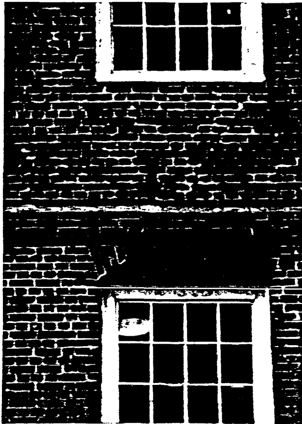
ILLUSTRATION 61. OLD STATE HOUSE: PATCHED CRACK IN NORTH WALL NEAR NORTHEAST CORNER, 1987.
