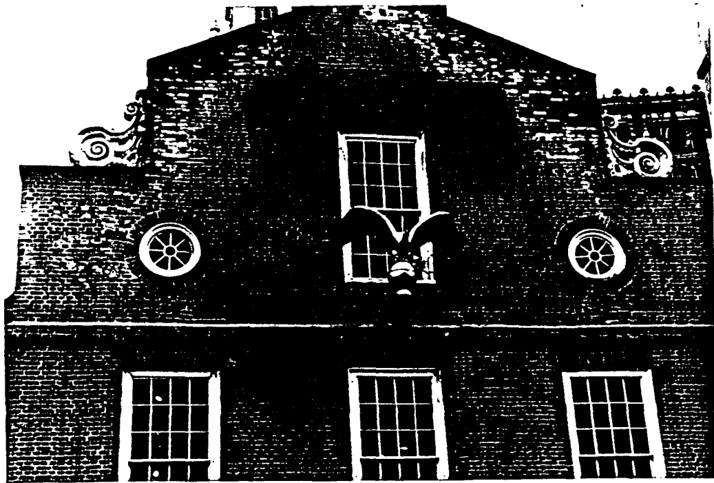
ILLUSTRATION 12. OLD STATE HOUSE: WEST WALL, PARAPET EFFLORESCENCE, 1987.
