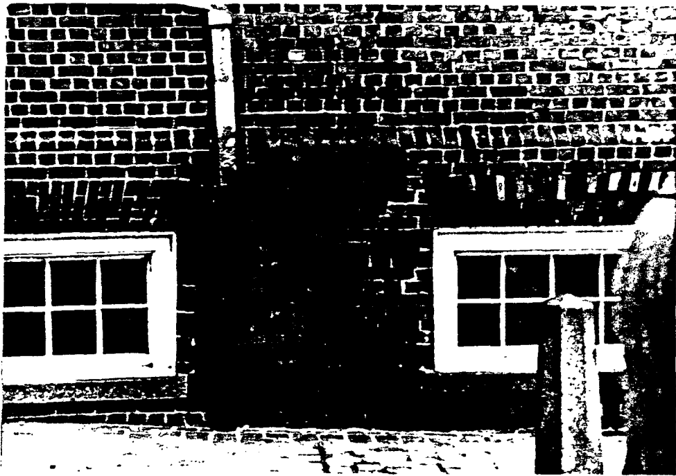
ILLUSTRATION 7. OLD STATE HOUSE: SOUTH WALL, WEST END, BRICKWORK NEEDING REPOINTING, 1987.
