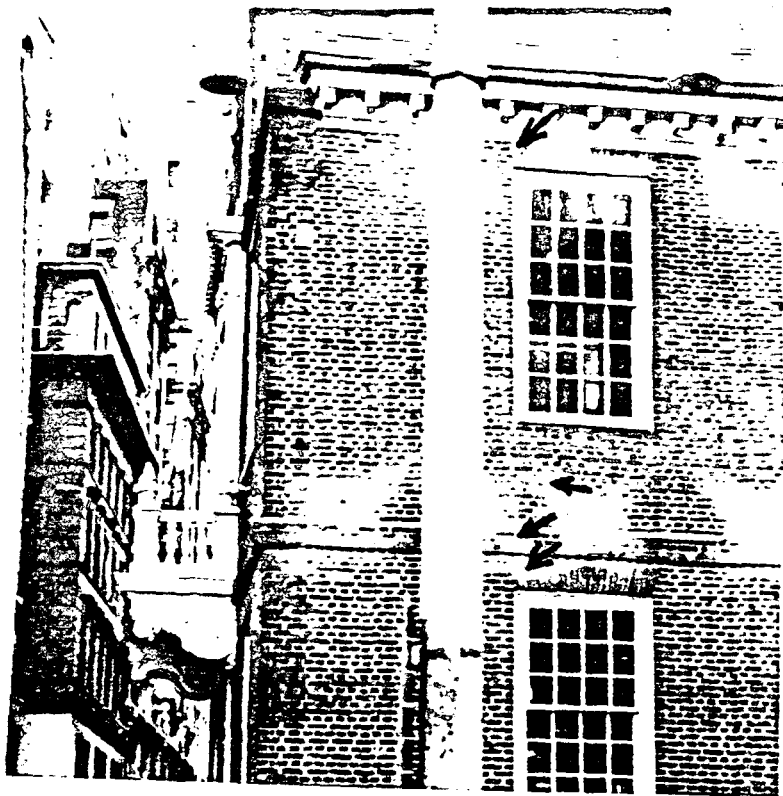
ILLUSTRATION 14. OLD STATE HOUSE: NORTH WALL, EAST END, CRACK IN BRICKWORK (FOLLOWS ARROWS), 1987.
