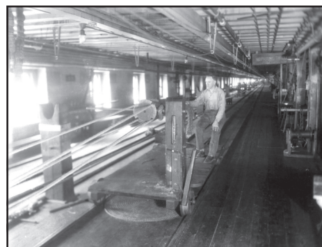
Until the 1950s, ropemaking required a facility as long as the rope being made. This ca. 1936 view of James Lee on one of the traveling carts gives an indication of the length of the Ropewalk, which made rope in lengths up to 200 fathoms (1,200 feet). (BOSTS-9541)
