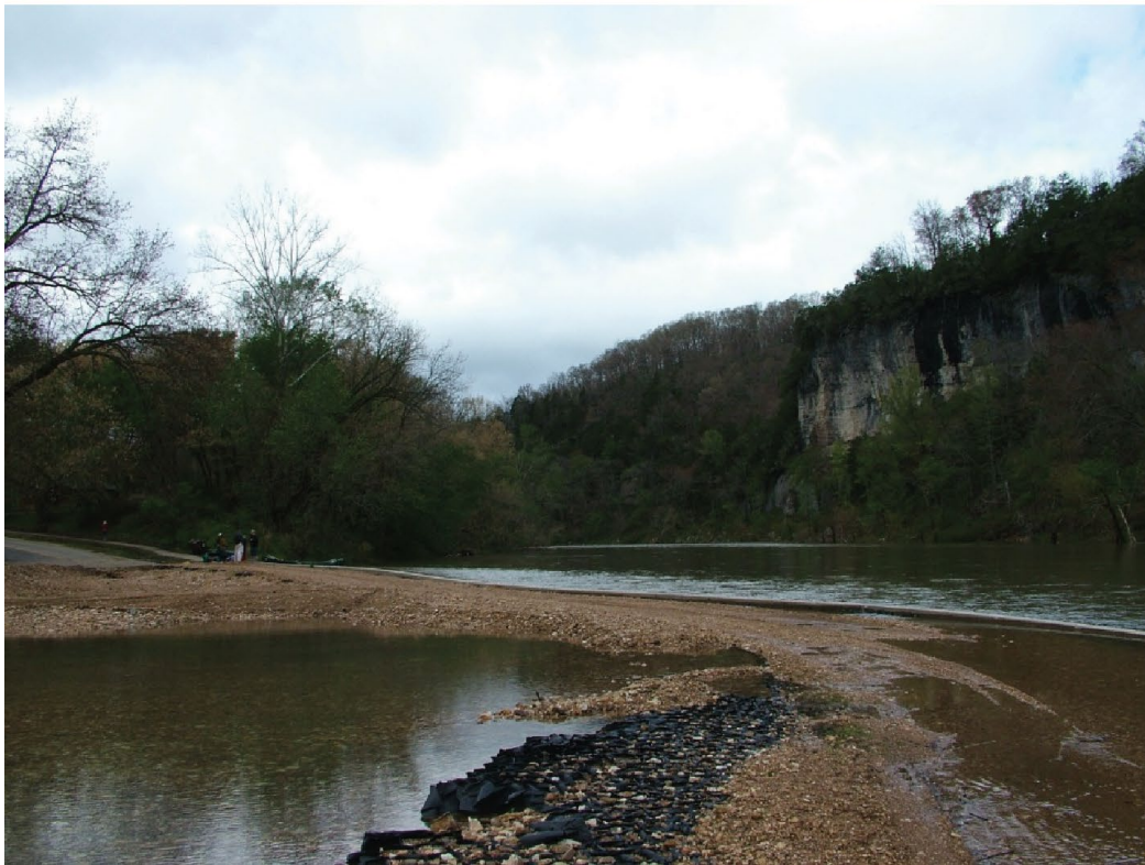
Figure 24. Photographs of shoreline-loss control structures along the Buffalo River. Photographs show the concrete retaining wall and geotech meshing, used to mixed success to maintain the gravel bar at the Tyler Bend launch point. The river tends to erode around the structures and wash them away or render them useless. Top photograph is looking upstream from the launch. Bottom photograph is looking downstream approaching the launch. Photographs by Andrea Croskrey (NPS Geologic Resources Division) taken in spring 2007.
