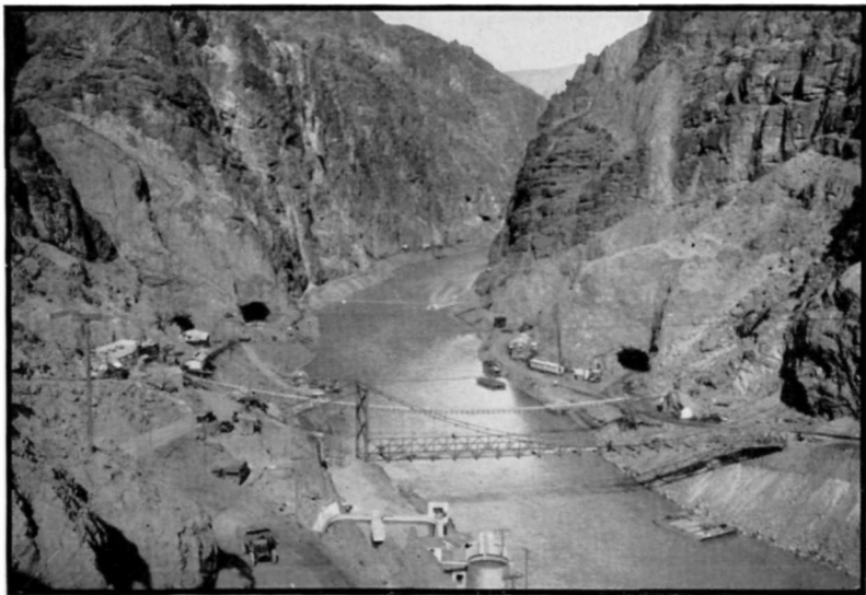
View Upstream February, 1932, Showing Tunnel Outlets
