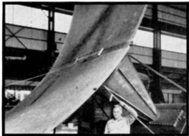
Taking X-Ray Photograph of Weld
