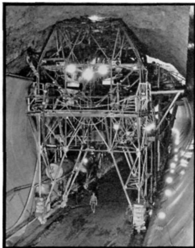
Arch Lining... Gun Carriage in Foreground
