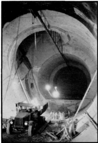
Intersection . . . Incline from Arizona Tower and Division Tunnel
