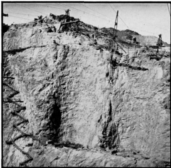
Completed Excavation for Nevada Intake Towers
