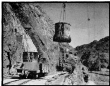
16 Tons Concrete in Transit to Dam
