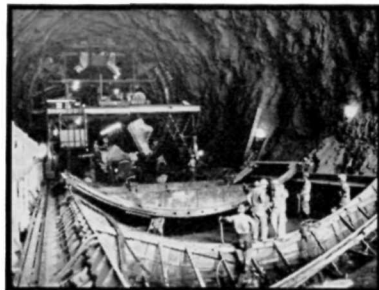
Lining Invert and Sidewall
