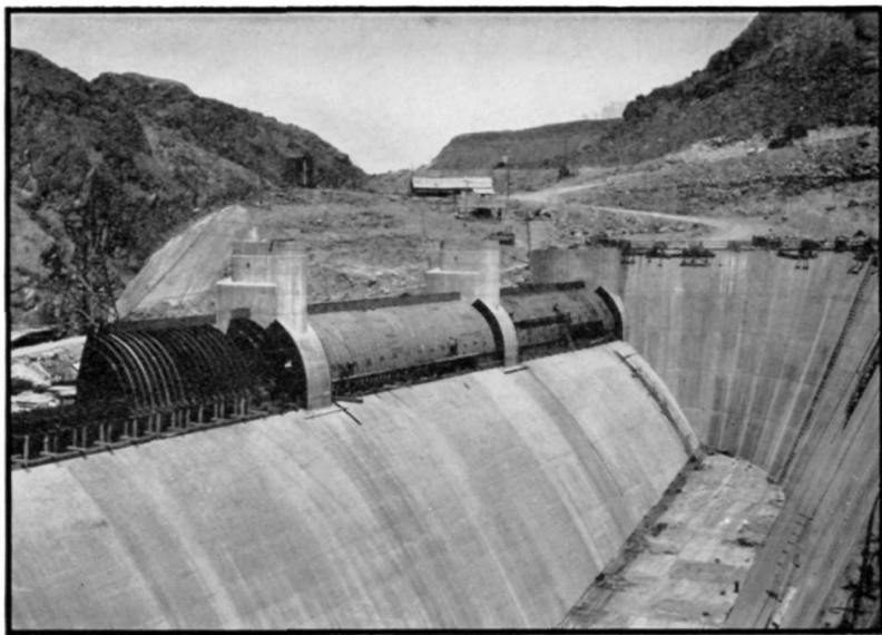
Arizona Spillway Showing Two Gates Installed
