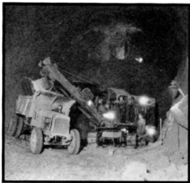
Excavating Penstock Header Tunnel
