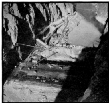
Building Upper Cofferdam
