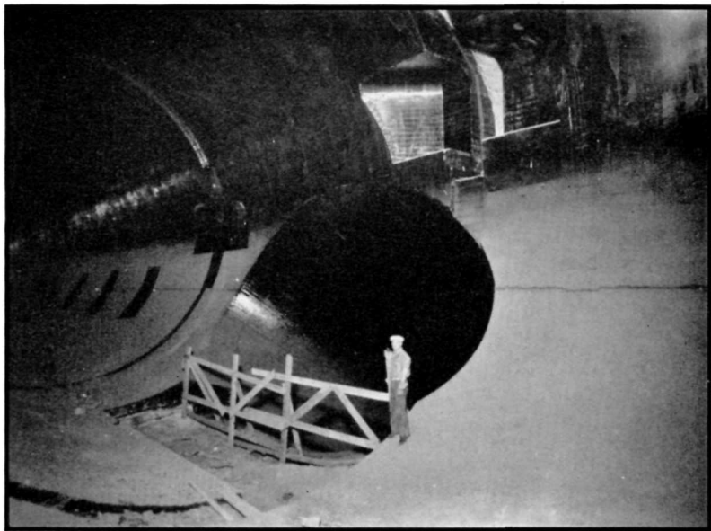
Intersection of Penstock and Penstock Header Tunnels
