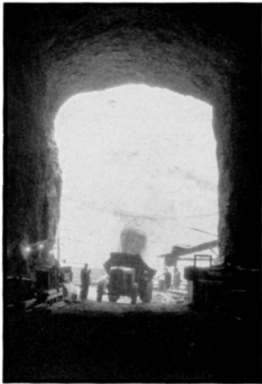
Arizona Construction Adit
