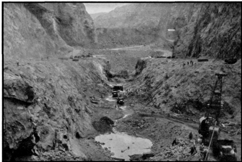
Dam Excavation Practically Completed
