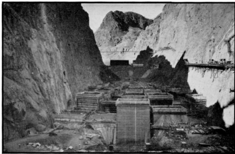
View Downstream September, 1933 . . . Note Cooling Plant and Tower on Lower Cofferdam
