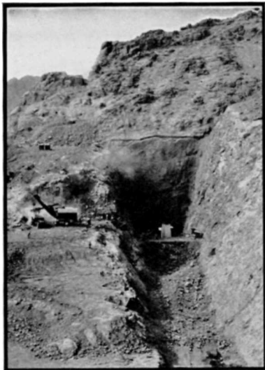
Excavation for Nevada Spillway Looking Toward Inclined Shaft
