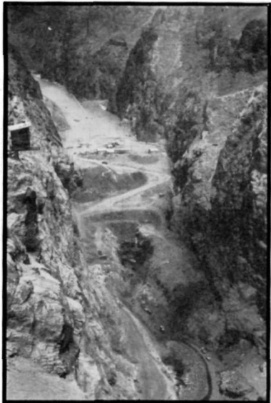
Excavation for Dam Foundation
