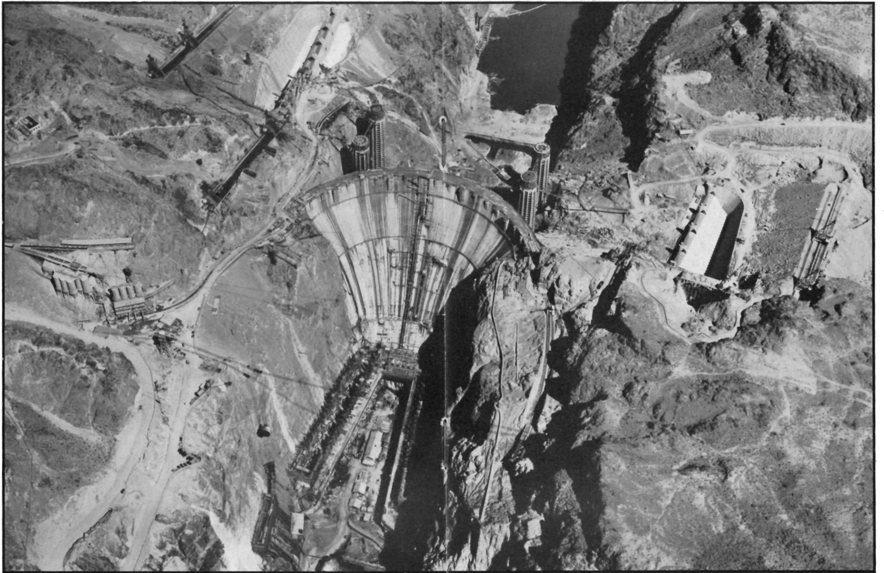
Aerial View of the Dam and Appurtenant Works at the Time of Initial Storage of Water in the Reservoir
