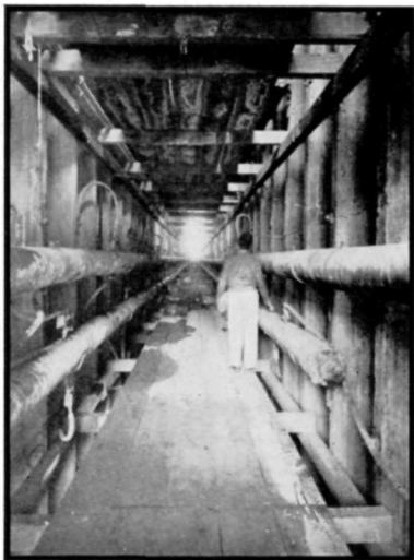
Slot Through Middle of Dam...Note Supply Lines for Cooling Pipes
