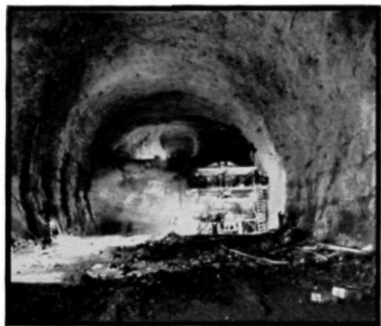
Drilling Jumbo at Tunnel Face
