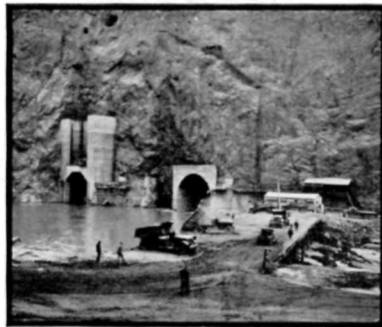
Building Temporary Dam for Diversion
