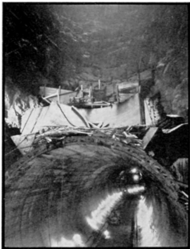
Intersection Nevada Spillway Shaft and Diversion Tunnel
