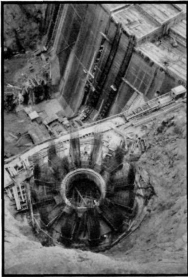
Looking Down on Nevada Tower
