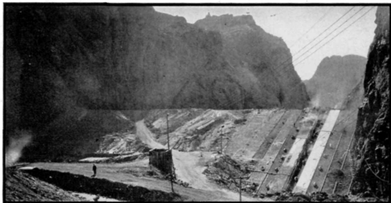
Completed Upper Cofferdam . . . View Downstream
