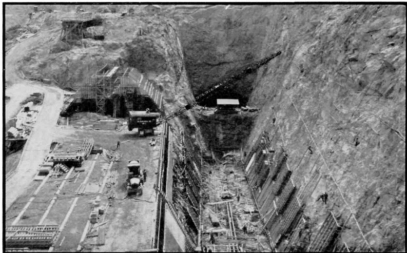
Lining Channel of Nevada Spillway
