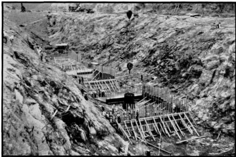
Pouring First Bucket of Dam Concrete
