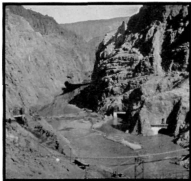
Temporary Dams in Place
