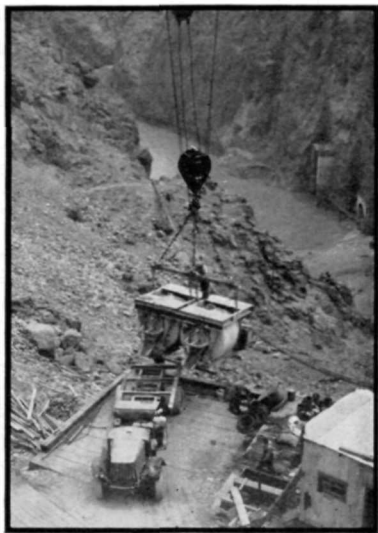
Load of Concrete
