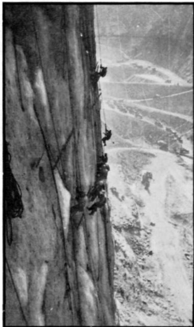
Scaling Above Power House
