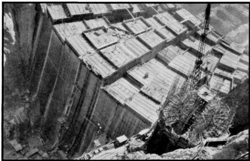
Upstream View of Dam When Approximately 300 Feet High, March, 1934
