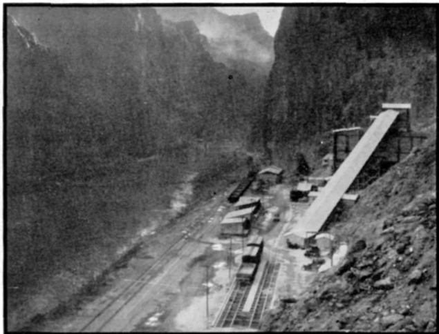
Low Level Concrete Mixing Plant
