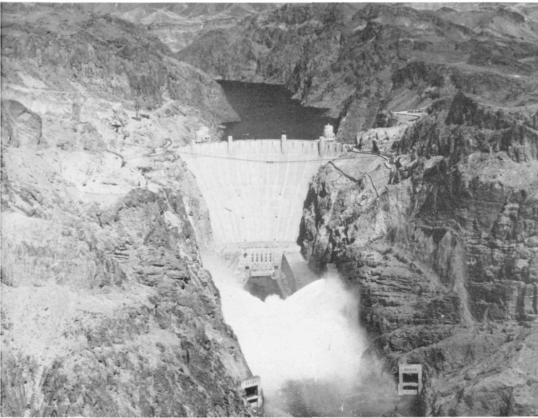
Boulder Dam's canyon wall outlets discharging a Niagara of water
