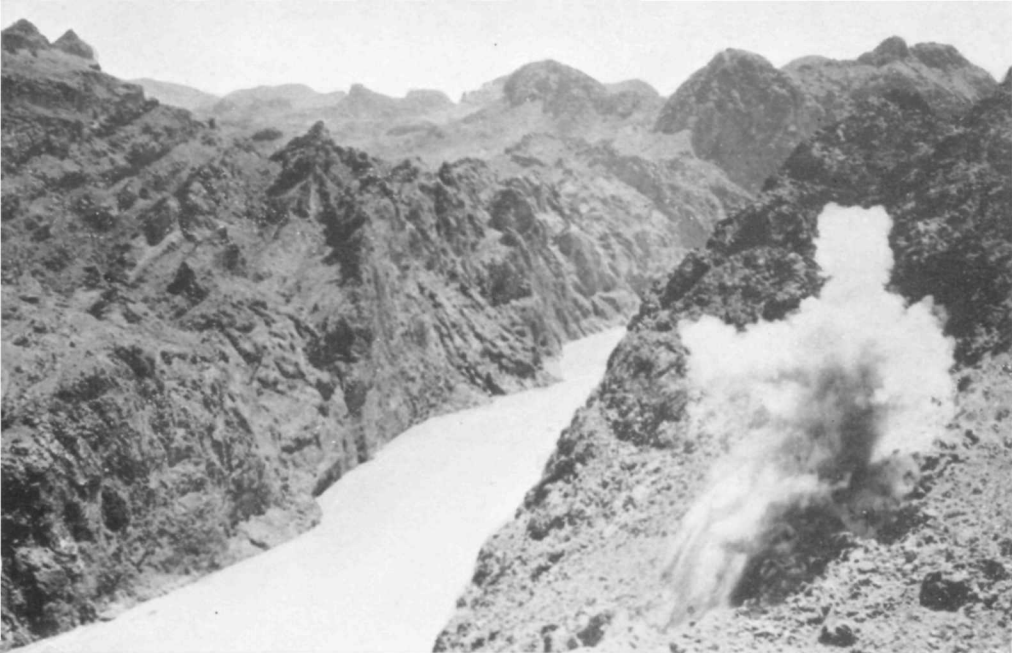
Blasting out the construction road to the dam site
