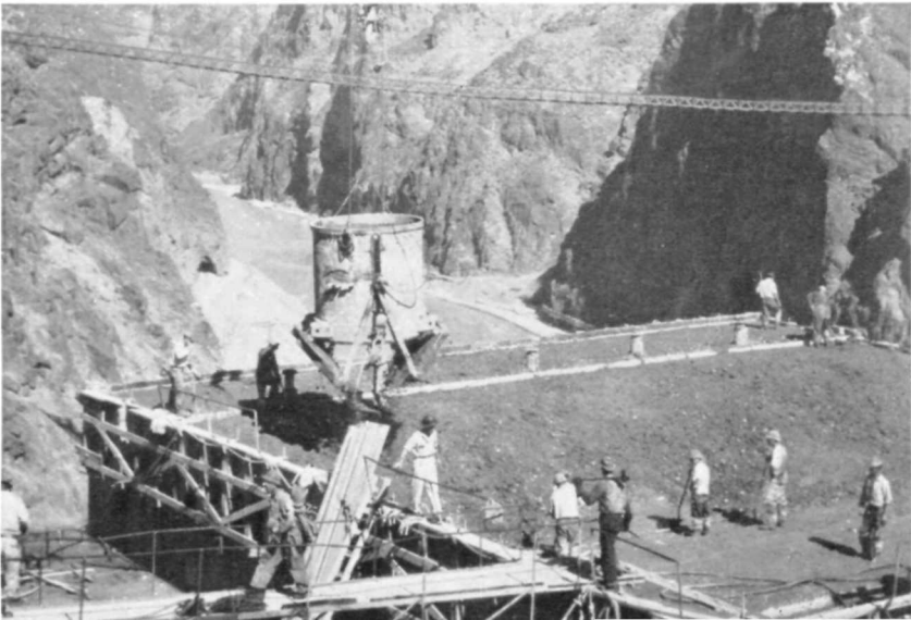
Dumping a bucket of 16 tons of concrete
