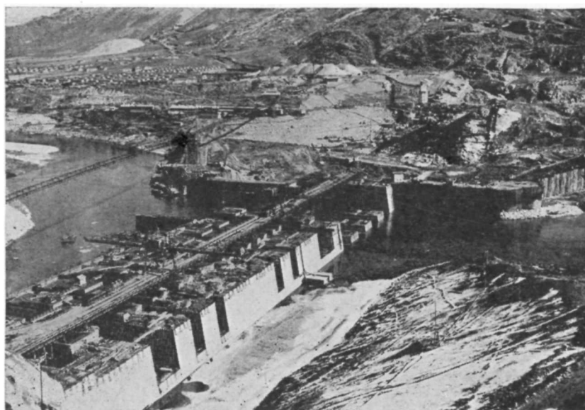
Block by Block the goliath dam takes form.
