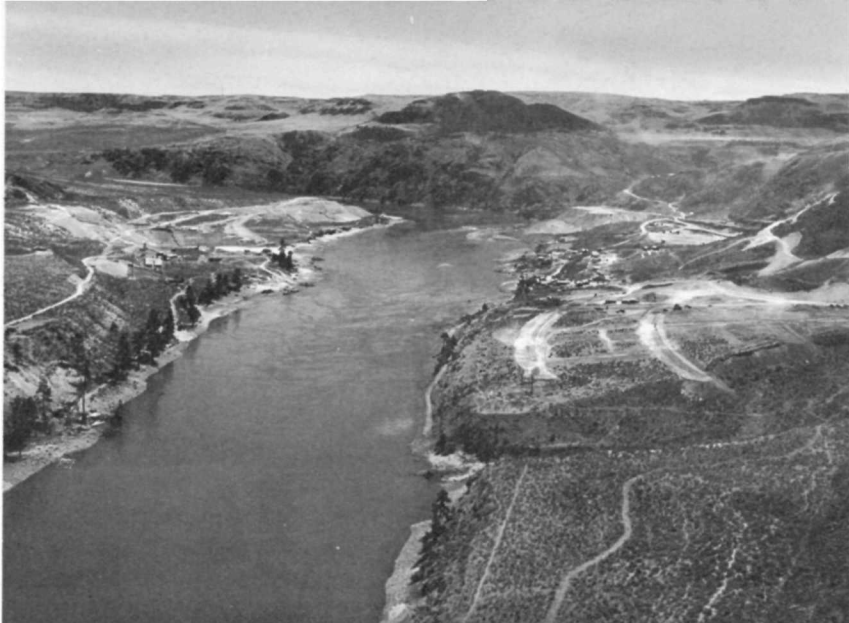
This is the site of Grand Coulee Dam as it looked before the first contract for its construction was let on July 13, 1934.
