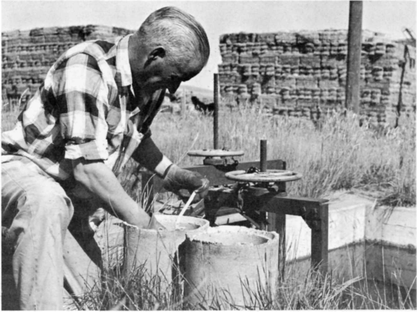
A ditchrider travels the project's canals daily, turning water into the farmers' ditches when needed and keeping an account of the amount of water used at each farm.
