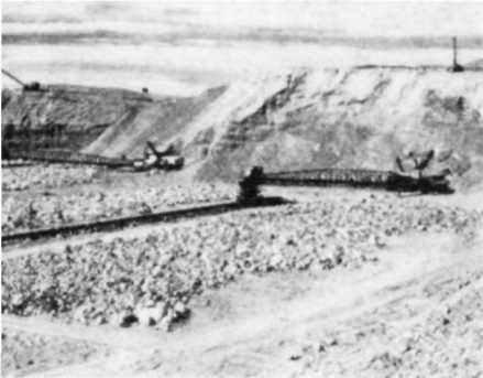
Electric shovels and belt conveyors move 25 thousand yards of pit-run sand and gravel in a day
