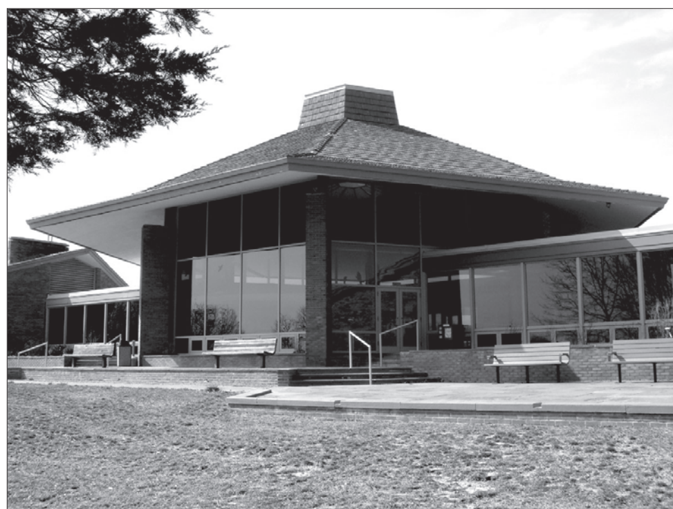
The modernistic Salt Pond Visitor Center (1965) was a clear departure from the traditional rustic architecture of parks. It has features typical of “Mission 66” visitor centers like views of the landscape through glass, separate wings for museums and theaters, and use of concrete, glass, and steel throughout. The building was found eligible for the National Register of Historic Places in 2000. (National Park Service photo)
