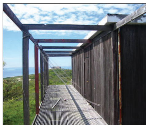
The Hatch House (1960) is nestled into a hillside on Bound Brook Island with sweeping views of Cape Cod Bay. Lightweight panels on the west wall shown here open up to the view with a simple pull of the ropes. (National Park Service photo)
