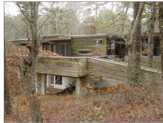
Reminiscent of Wright’s Falling Waters , the Kugel-Gips House exhibits classic Modern house characteristics: flat roof, open floor plan, expansive windows, and intimate connection with the outdoors. (National Park Service photo)
