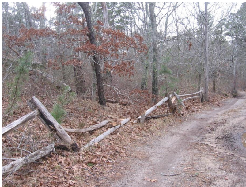
Split rail before repairs
