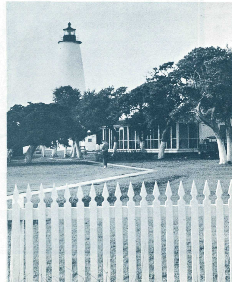
Ocracoke Lighthouse—oldest on the North Carolina coast
