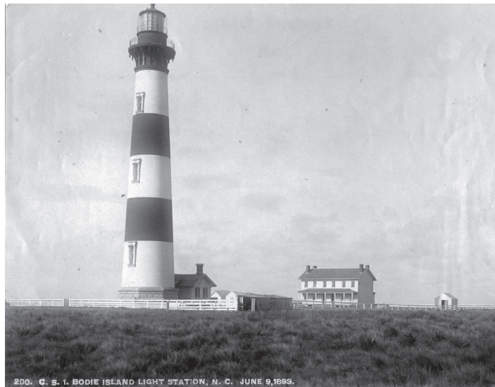
The Bodie Island Lighthouse has changed little since this photo was taken in 1893.
