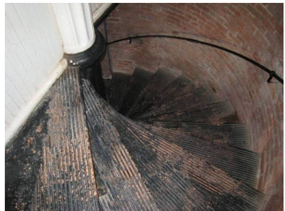
Figure C-72 Original cast-iron steps leading down from Seventh Floor Landing.
