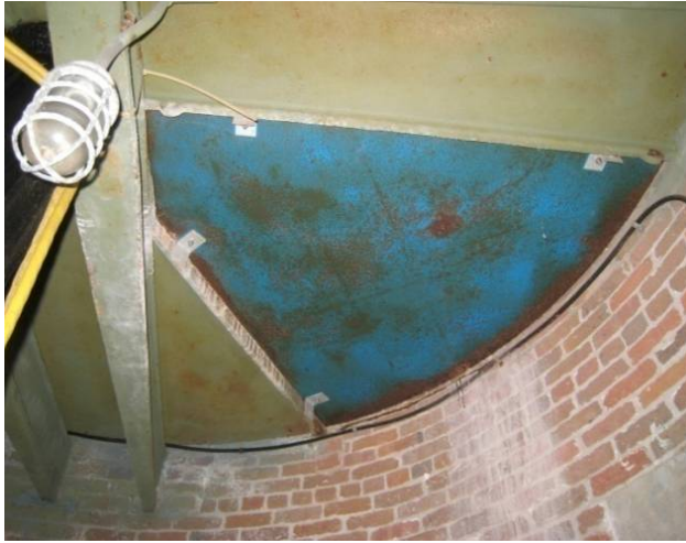
Figure C-44 Modern replacement floor plate at Second Floor landing.
