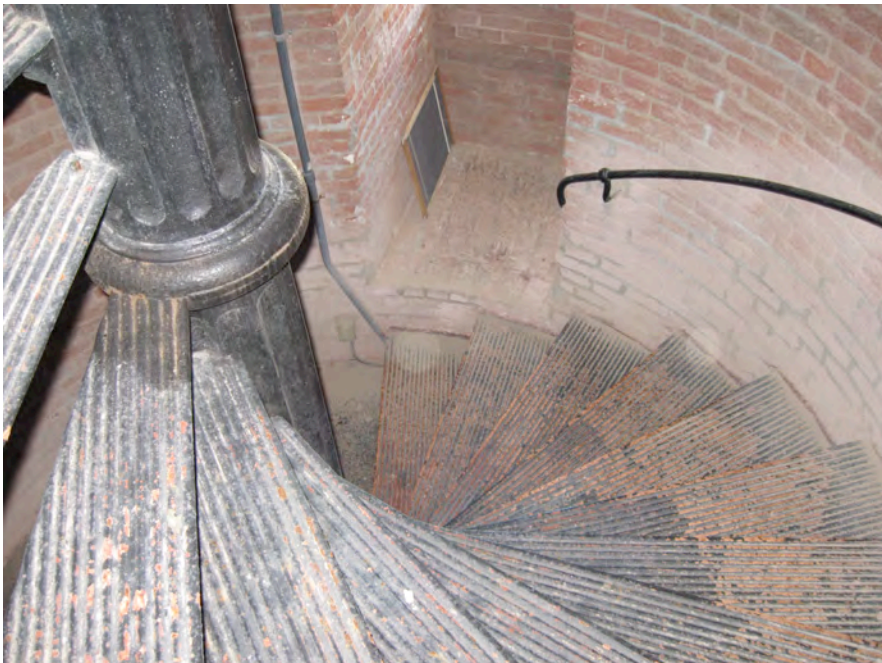
Figure 2. Cape Lookout Lighthouse, September 2008. This photograph shows typical interior features, including the exposed brick walls and cast iron spiral stair. Photograph by author.
