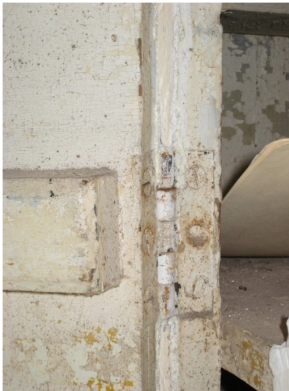
Figure C-94 Cabinet's five-knuckle hinge and batten.
