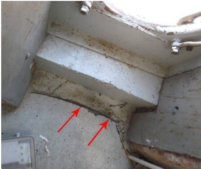
Figure C-85 Jacking of iron floor plate at doorway to Observation Deck.
