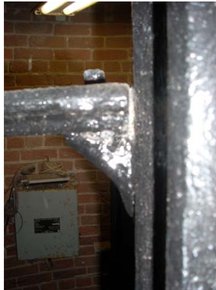
Figure 3 – Pin Connection at Interior Support Column
