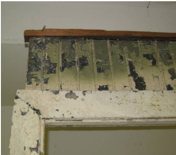
Figure C-49 Close-up view of salvaged wall plate, board wall and door casing
