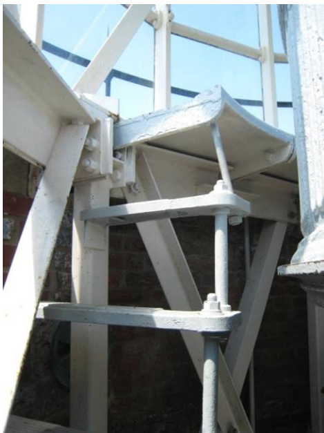
Figure C-101 Original cast-iron ship's ladder connecting to Lantern floor plates.
