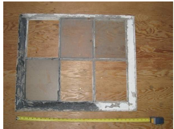
Figure C-39 Exterior exposure of lighthouse window sash in the collection of the North Carolina Maritime Museum.
