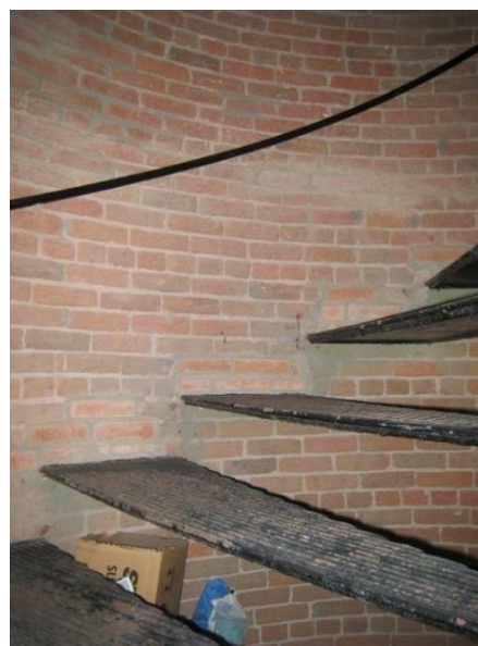
Figure C-62 Typical cast-iron treads of Spiral Staircase.
