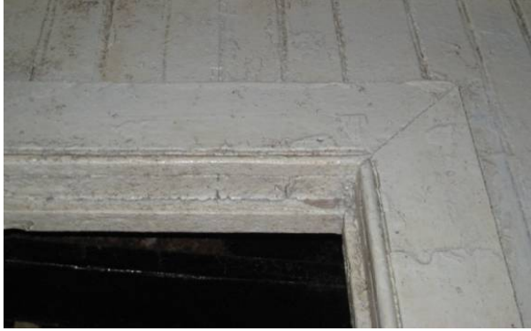
Figure C-79 Seventh Floor door casing. Note miter cut of corner.
