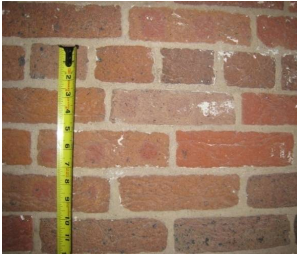
Figure C-9 Brickwork of interior face of core wall.
