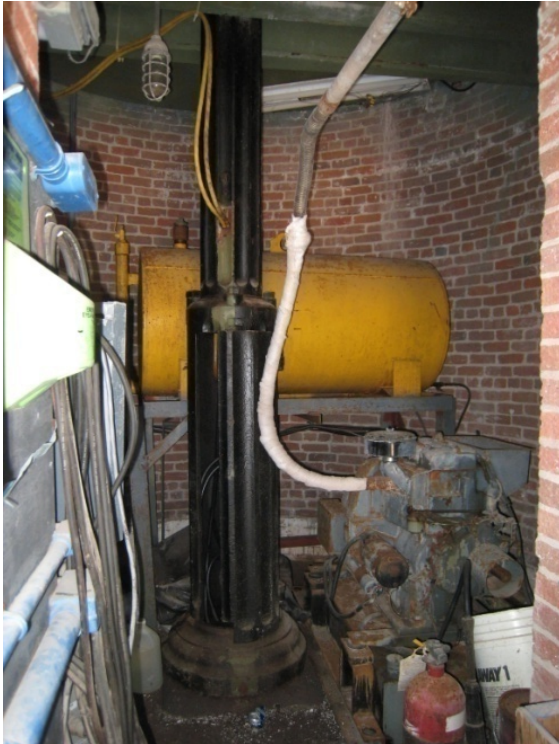
Figure C-56 View of First Floor Room from Passageway.
