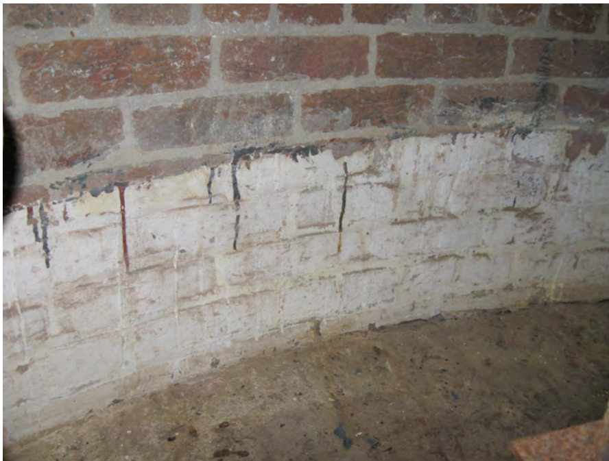
Figure 12. Cape Lookout Lighthouse, September 2008. Additional evidence of limewash was found in the boiler room, in an area previously covered by a wood platform. Photograph by author.
