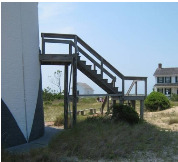
Figure C-35 Stairs for Main Entrance.
