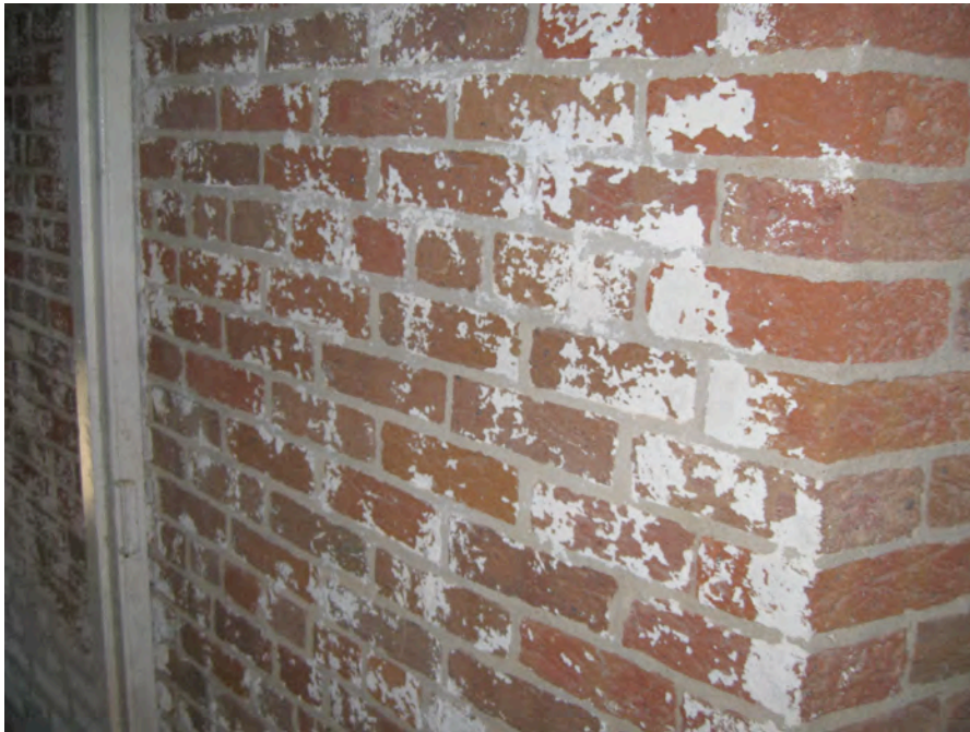
Figure 11. Cape Lookout Lighthouse, September 2008. Evidence of white limewash on the entry vestibule walls. All other finishes have been removed from the interior brick walls. Photograph by author.
