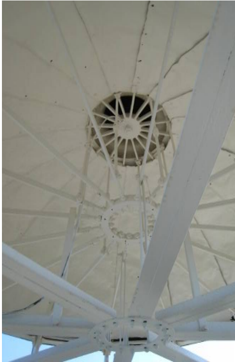
Figure C-17 Structural supports and central ventilator of dome.
