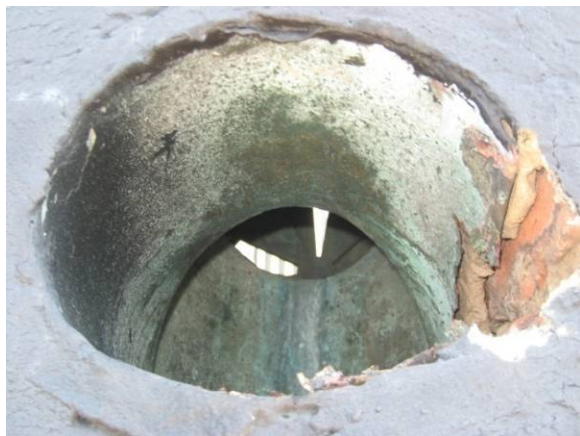
Figure C-11 Natural cement bedding mortar exposed at Watch Room air vent.
