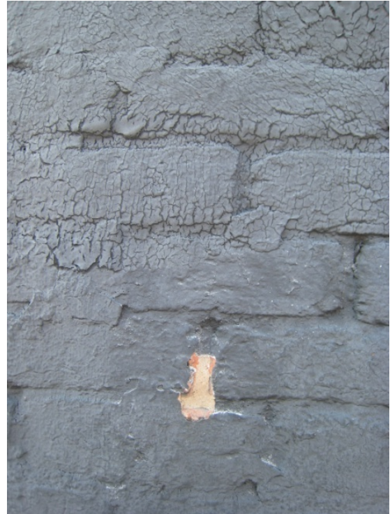
Figure C-108 Non-breathable coating on exterior masonry.
