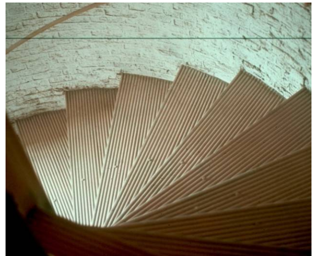
Figure C-47 Spiral stair and masonry finishes, 1976-1981 photograph. (CALO Coll.)
