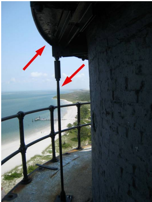
Figure C-18 1989 steel reinforcement of Gallery deck and connecting rod.
