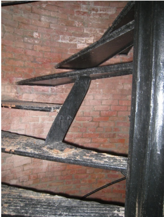
Figure C-73 1914 tread modification to accommodate the weight for oscillating mechanism.
