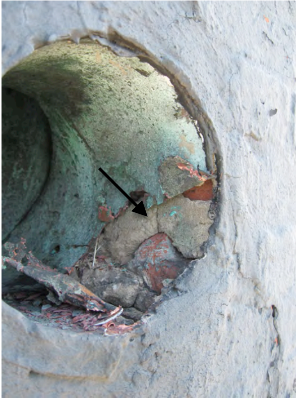
Figure 3. Cape Lookout Lighthouse, September 2008. Location of well-preserved original mortar that was sampled for analysis. Photograph by author.
