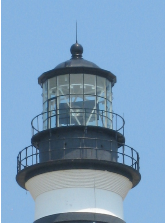
Figure C-21 Lantern, Lantern Gallery and Watch Level Observation Deck.
