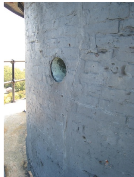
Figure C-26 Exterior view of one of four Watch Room air vents.
