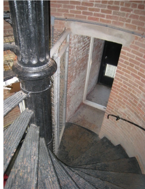
Figure C-64 Second Floor entrance passageway, spiral stairs, and modern steel fence enclosure.
