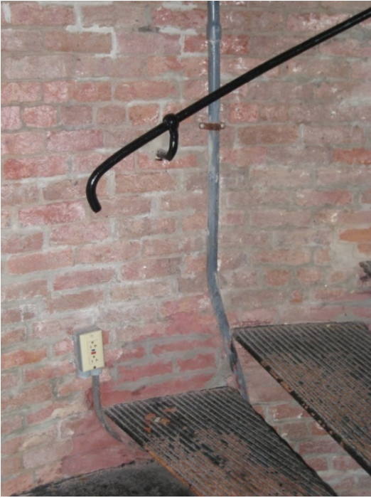
Figure C-46 Original iron handrail of 1-inch diameter.
