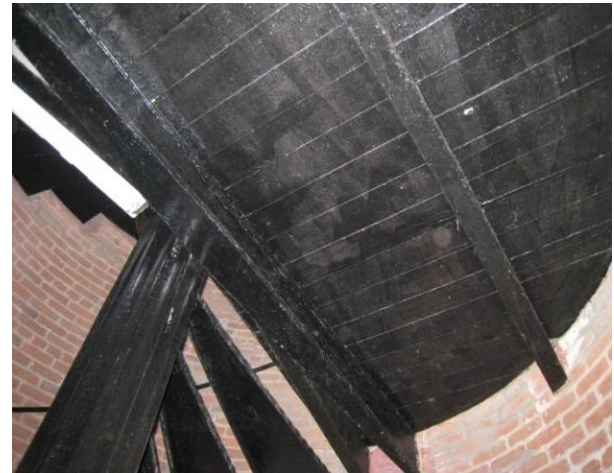
Figure C-66 Third Floor wood Landing.
