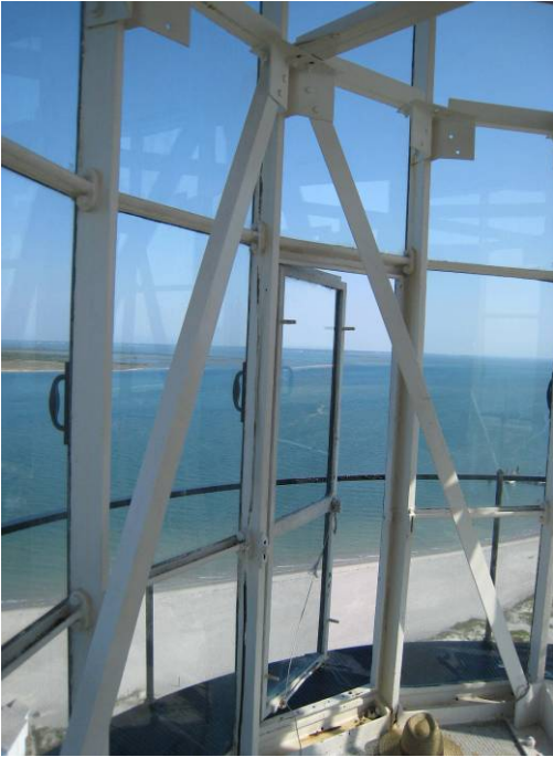
Figure C-31 Doorway to Lantern Gallery.
