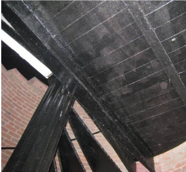
Figure C-15 Wood deck and floor joists of rebuilt 1867 Third Floor landing.
