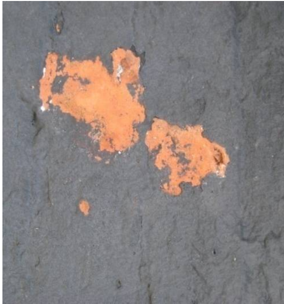
Figure C-37 Physical evidence of red limewash on tower's exterior masonry.
