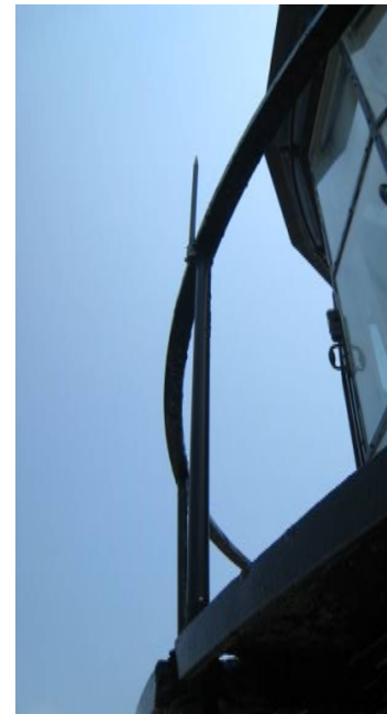
Figure C-36 Modern lightning rod at Gallery railing.
