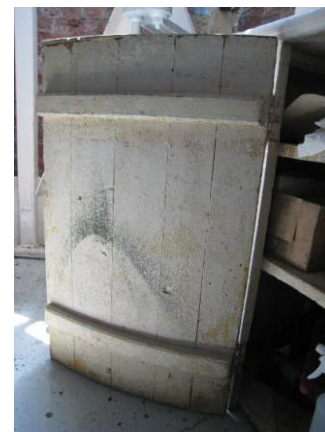
Figure C-92 Curved interior face of board-and-batten cabinet door.
