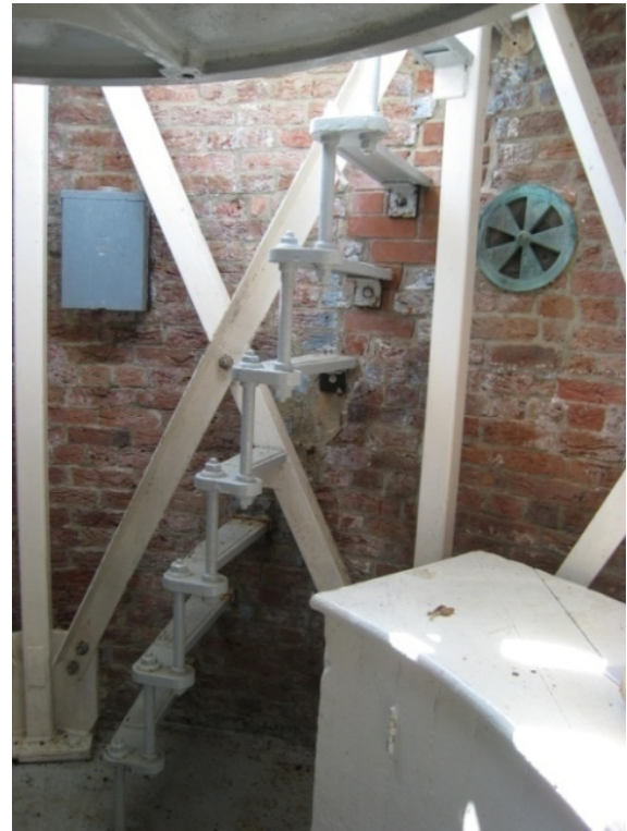
Figure C-89 Original cast-iron ship's ladder to Lantern.
