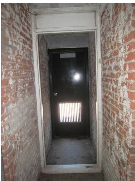
Figure C-61 Modified original exterior doorway and c.1914 interior door/transom framing in foreground.
