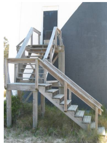
Figure C-29 Modern entrance stair to Second Floor
