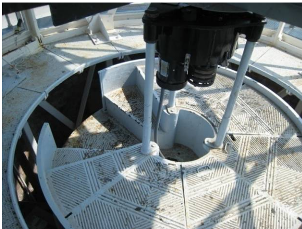
Figure C-97 Center cast-iron platform for beacon.
