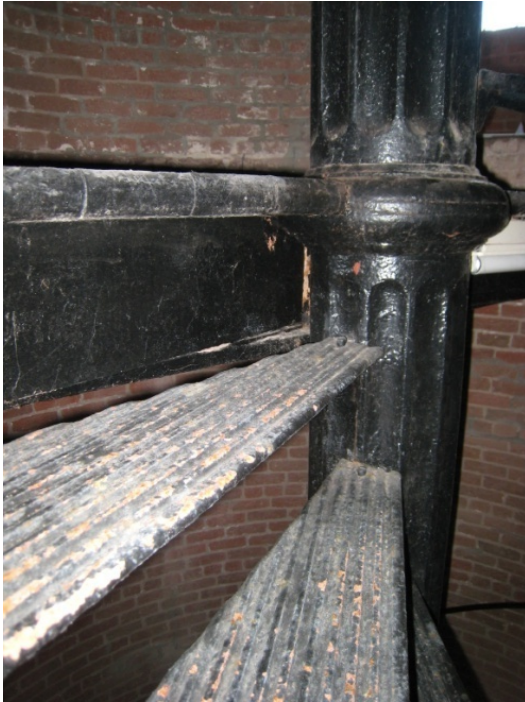
Figure C-67 Detail of bull nose edging of Third Floor landing.
