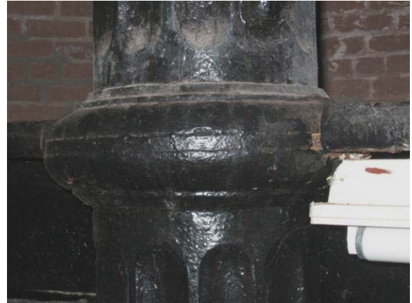
Figure C-14 Bolted connection between column sections.
