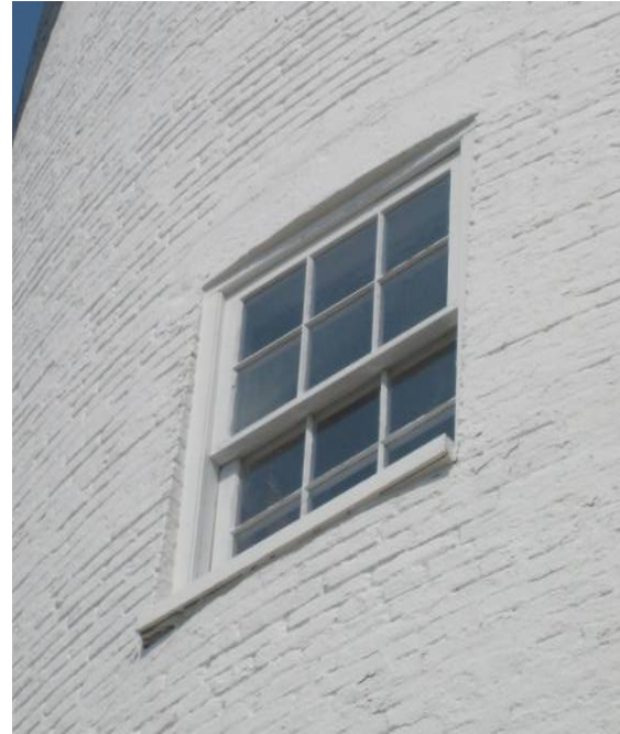
Figure C-32 Typical replacement window unit.
