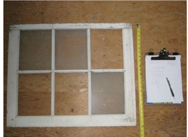
Figure C-50 Interior face of salvaged lighthouse window sash in North Carolina Maritime Museum.
