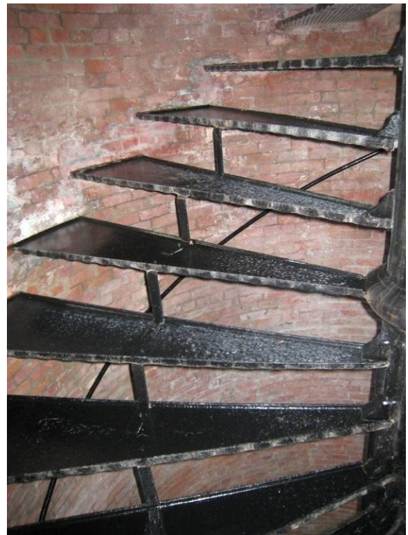
Figure C-74 Metal strap reinforcement of unknown installation date.
