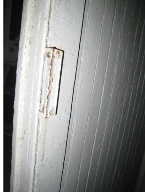
Figure C-81 Door latch keeper matches rim lock of extra door in North Carolina Maritime Museum collection.
