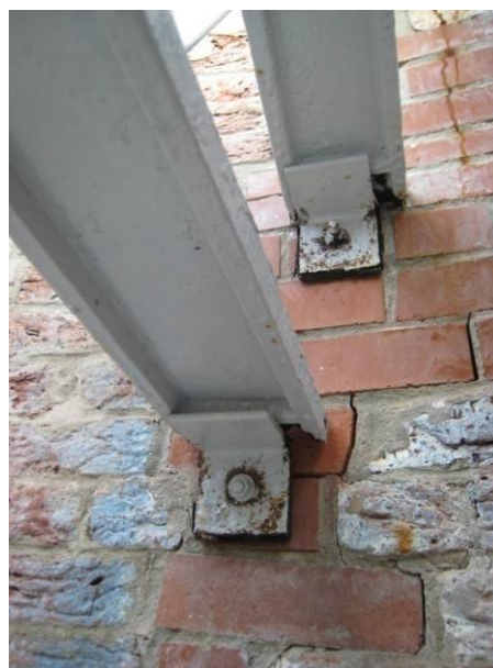
Figure C-8 Modern masonry repairs in Watch Room.
