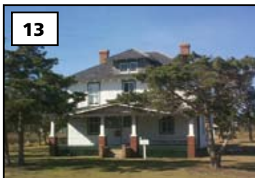
13 Theodore and Annie Salter House: serves as a visitor center; inside are exhibits and public restrooms.
