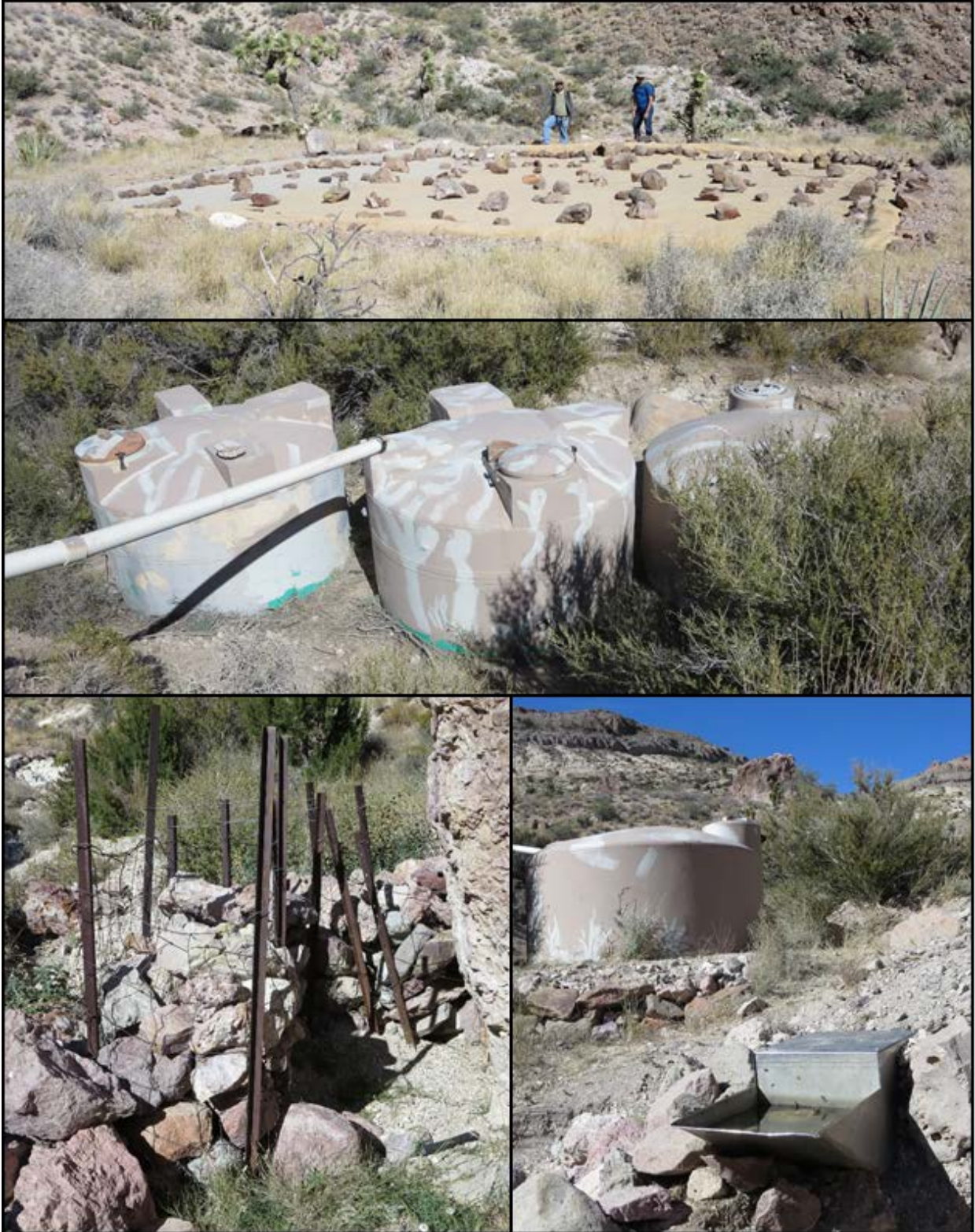
Figure 2. Kidney Spring. Top: Rainwater collector above tanks. Middle: Three tanks with pipe from rainwater collector. Bottom left: Gabion enclosing dry spring source. Bottom right: Drinker full of water below tanks.
