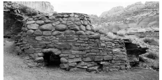
Lime kiln along Sulphur Creek.
